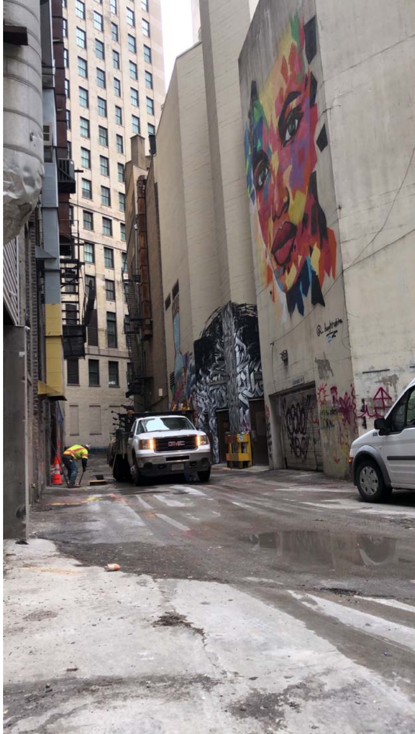
Photograph 2: View of Meade installing corrosion protection in alley
