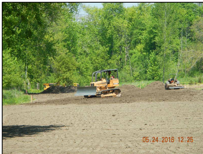
Clean soil being backfilled at a Tittabawassee River property.
