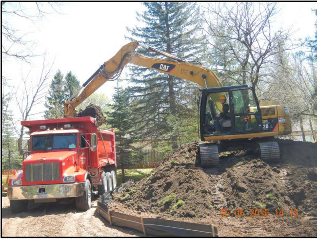
Loading contaminated soil into a truck for transport.
