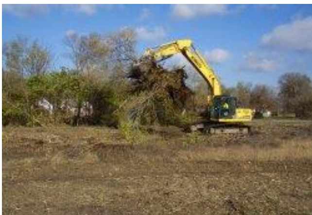
Earth-moving equipment clearing vegetation from the site.
