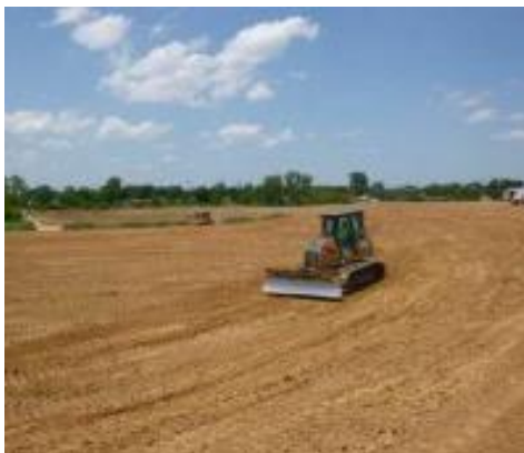
Placement of cover.
