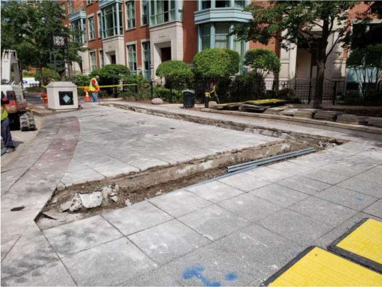
Overall site, looking northeast
