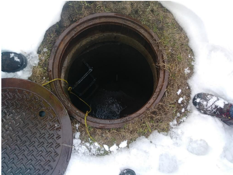
Photo 7: Mixing tank near treatment trailer
