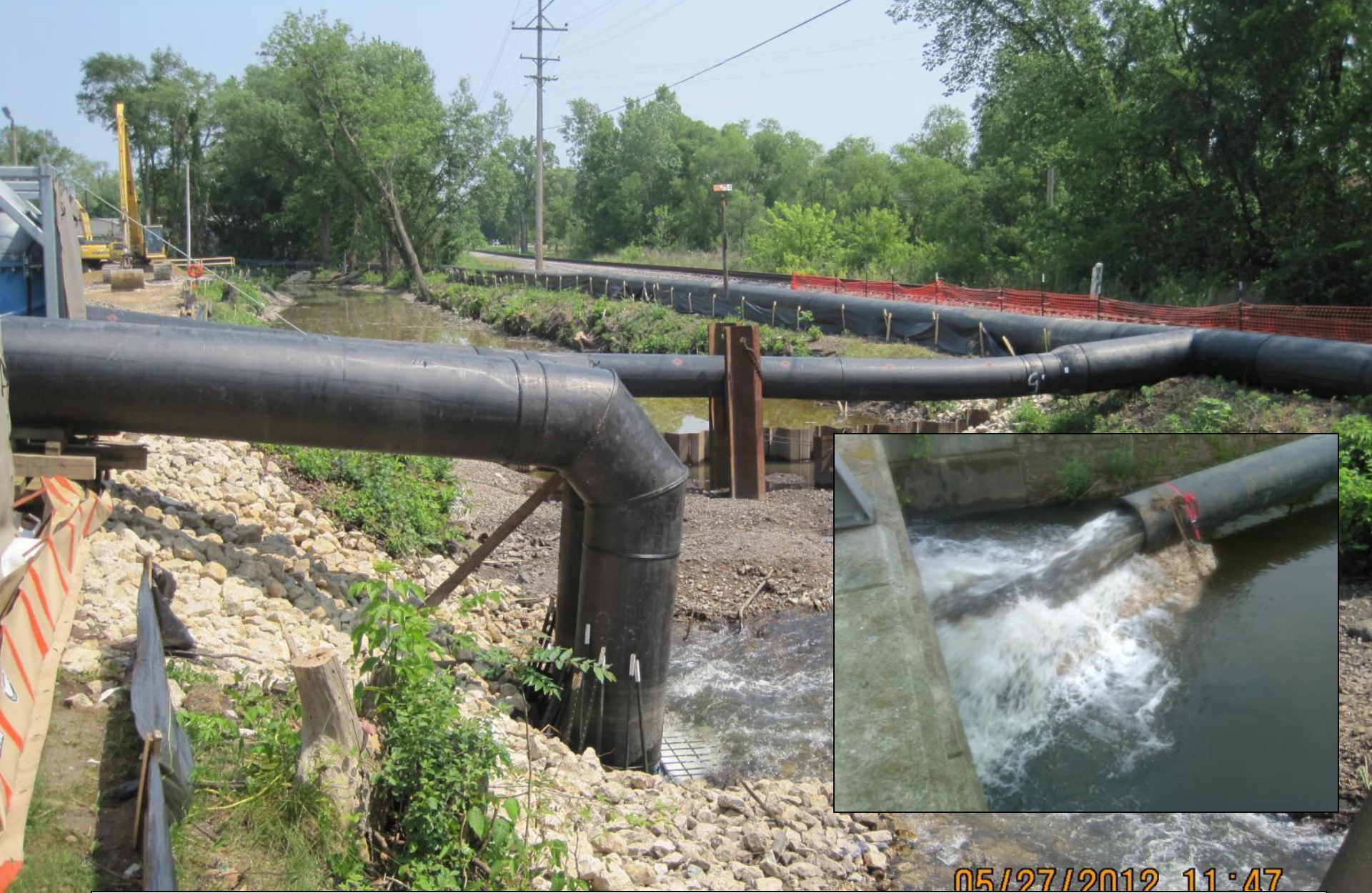
Creek Bypass Pump System
