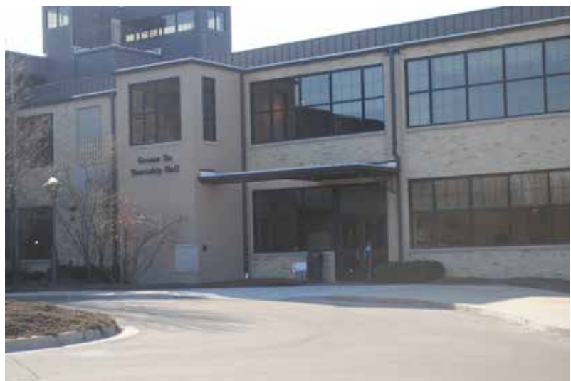
Grosse Ile Township building.
