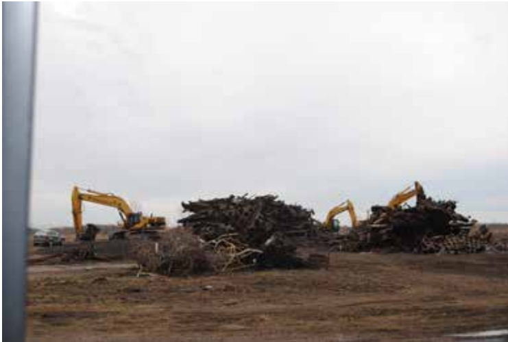
Teardown work at the site in March 2019.
