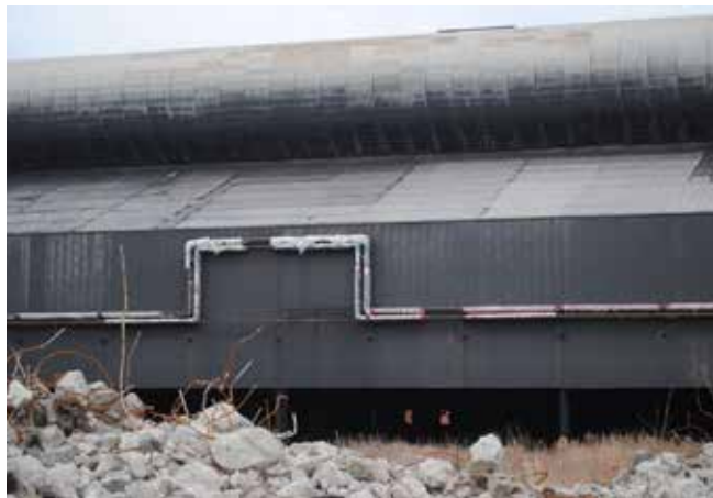
Pipe wrap across a building on the property.
