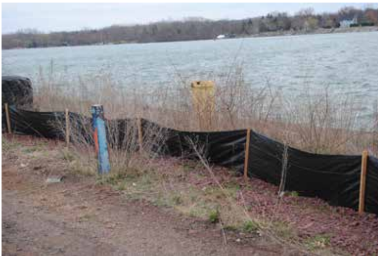
Silt fencing at east end of property by the river.
