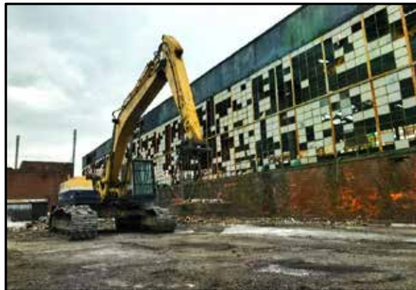
Teardown work at the site in April 2019.
