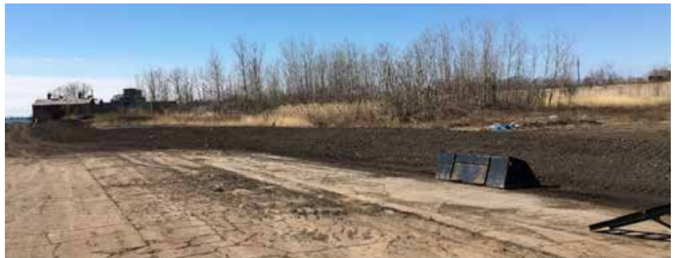
MSC installed an asphalt berm to reduce stormwater runoff to the Detroit River.
