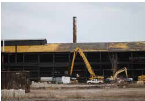
Building demolition began in January 2019.
