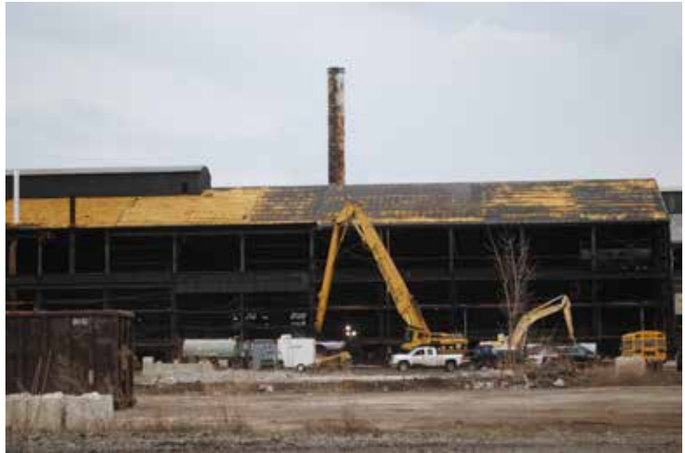
Teardown work at the site in March 2019.
