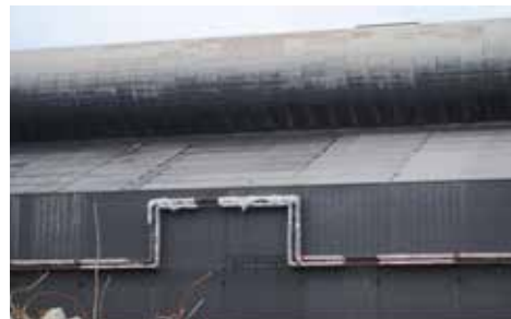
Asbestos-wrapped pipes.
