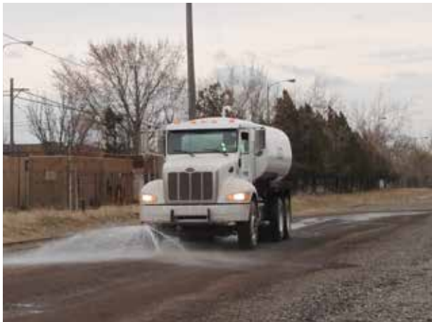
Trucks wet down the site to control dust.
