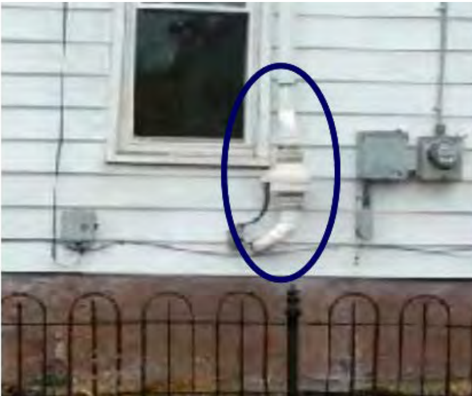
This photograph shows a vapor mitigation system installed on the outside of a house.
