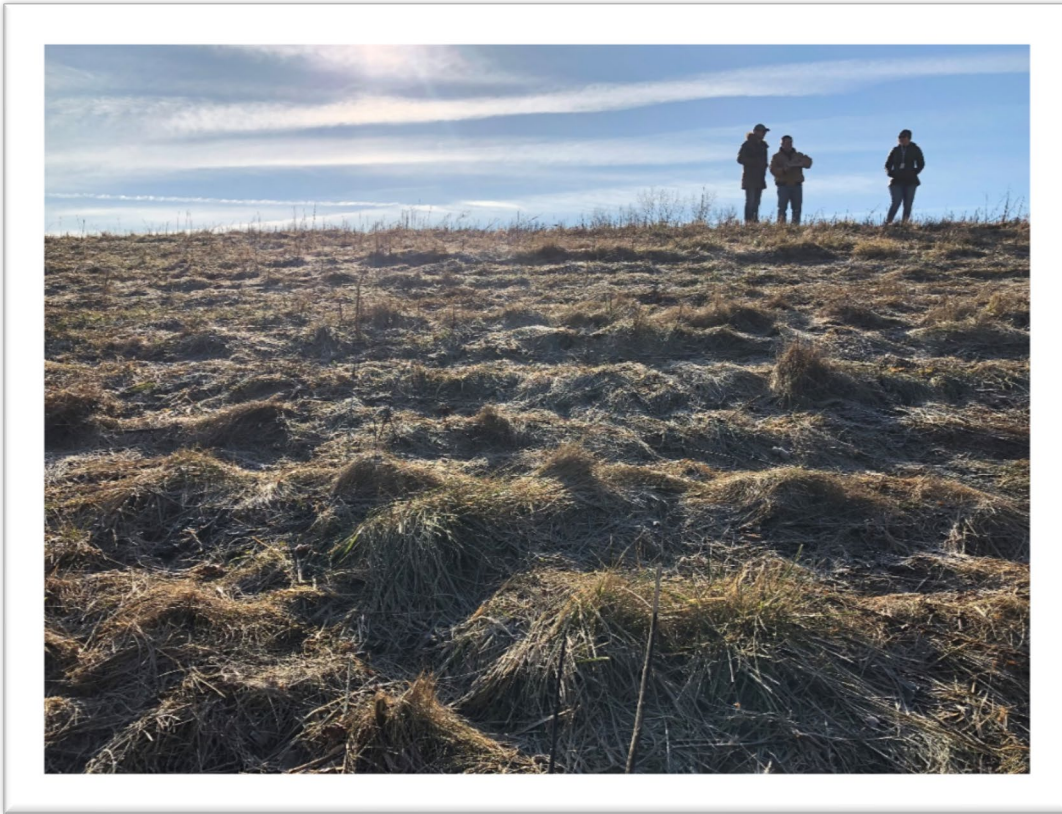
Photo 9: Grading along the northern portion of the cap, looking south.
