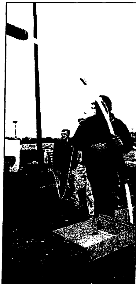
Ports and packers are placed exactly where needed immediately prior to installation
