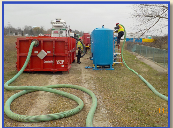
Vacuum removal of liquid granular activated carbon.
