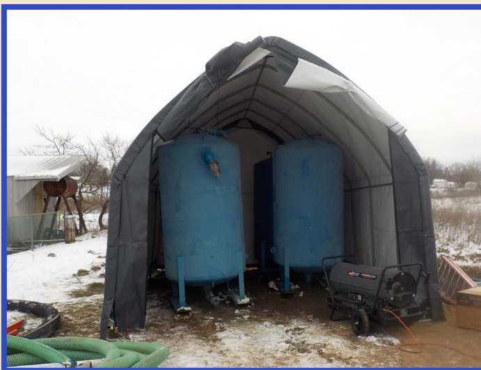
Warming liquid granular activated carbon prior to removal from treatment vessel.
