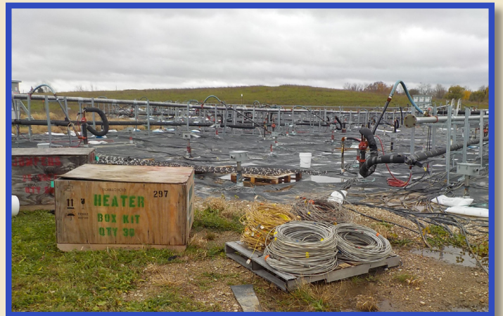
Demobilizing Area 1 ISTT well field components.
