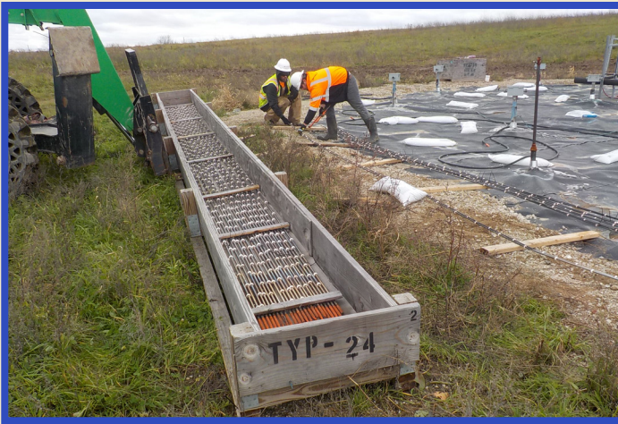
Removal and crating of ISTT heaters.
