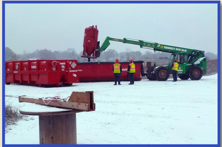
Transferring spent granular activated carbon to roll-offs for disposal.
