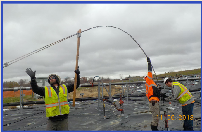
Removing ISTT heaters.
