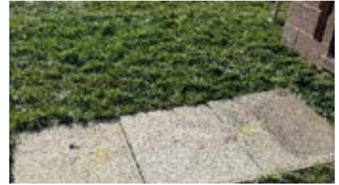
New sod is placed to restore yard.
