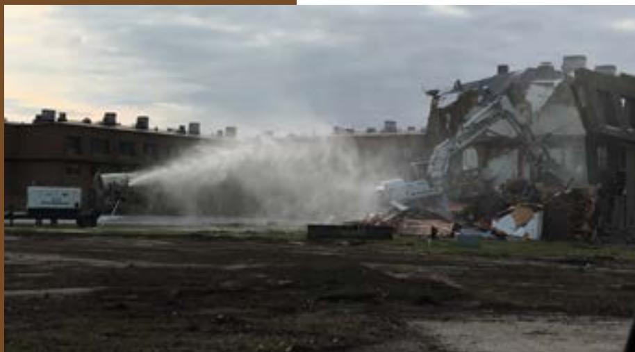
During demolition crews sprayed water to help keep down the dust.
