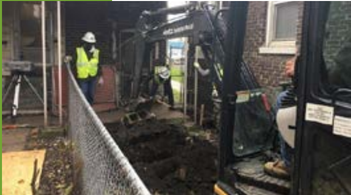
Contaminated soil is dug up and removed from yard.
