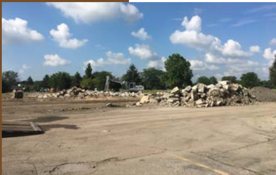
Demolition of Zone 1 nears completion.
