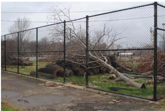
Fencing and vegetation has already begun to be moved at the site in preparation for the cleanup.
