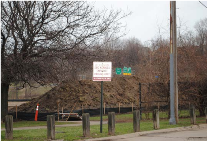
Work on the Towpath Trail extension is already visible. Here preparation is beginning on the foundation of a bridge.
