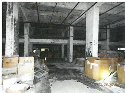
DSCN0055 – Central warehouse.
