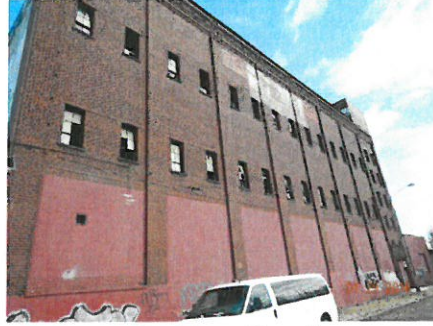
Front of building off Neville Ave.
