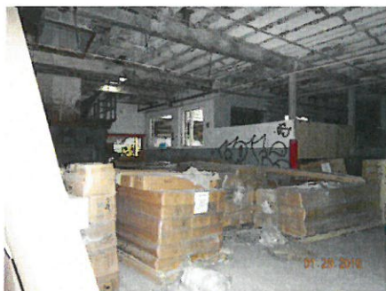
DSCN0058 – Central warehouse.
