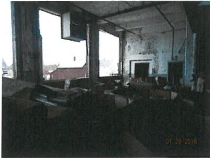
DSCN0064 – North warehouse open windows.
