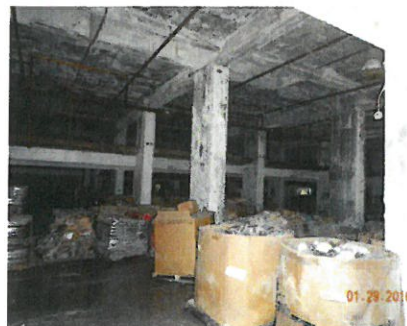
DSCN0056 – Central warehouse
