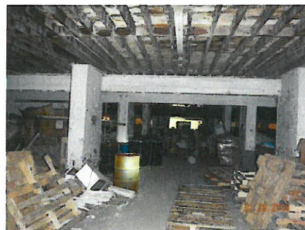
DSCN0070 – Central warehouse area.
