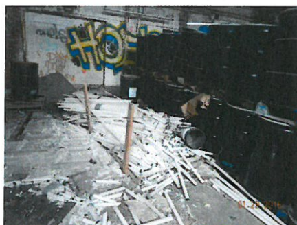
DSCN0049 – Southeast warehouse with drums of broken bulbs.
