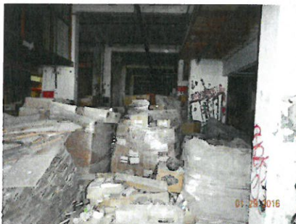
DSCN0020 – Central warehouse.
