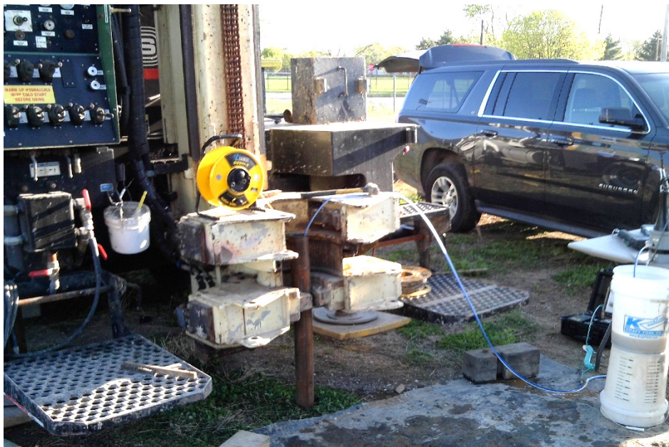
EPA monitors and takes samples of groundwater at the Elm Street site.
