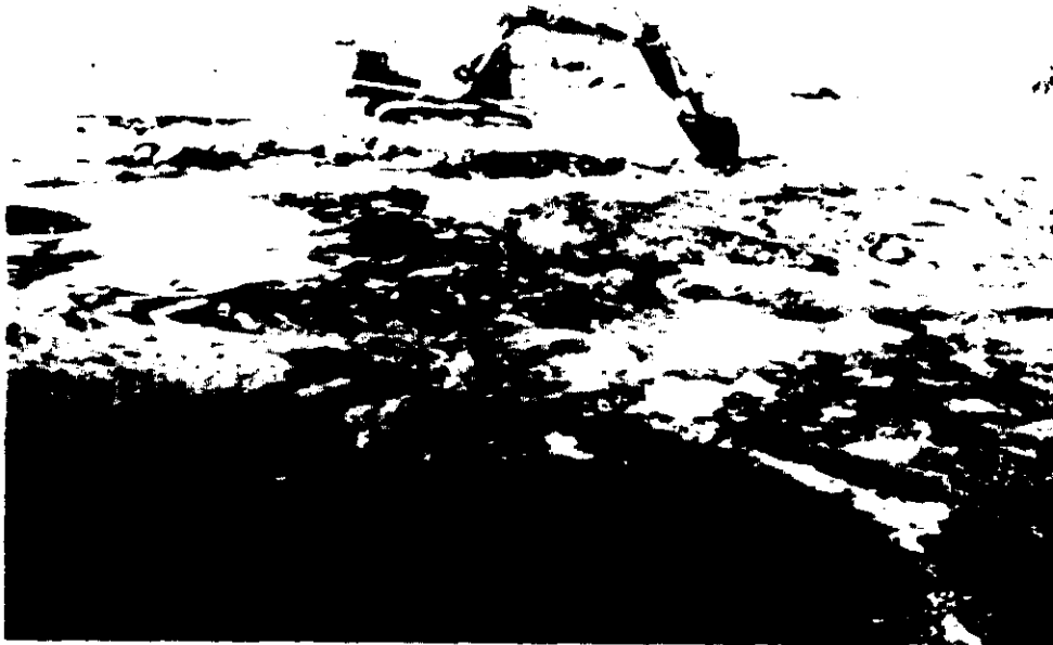
Figure 6-3. In-situ mixing with a backhoe at a large site. (Courtesy Albert H. Halff Associates)
