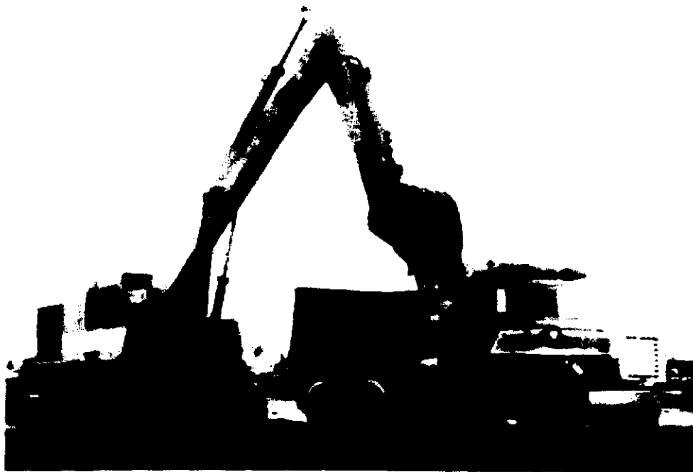
Figure B-7. Backhoe-dump-truck operation for removal of contaminated soils (Courtesy Albert H. Halff Associates).
