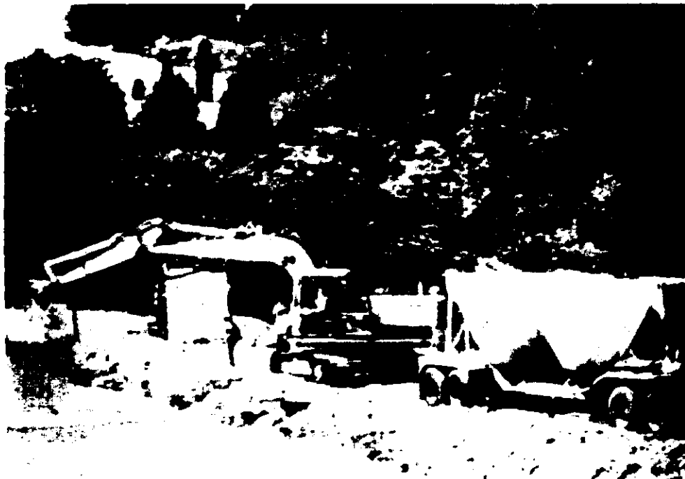
Figure 6-5. In-situ mixing equipment (Courtesy American Resources Corporation).
