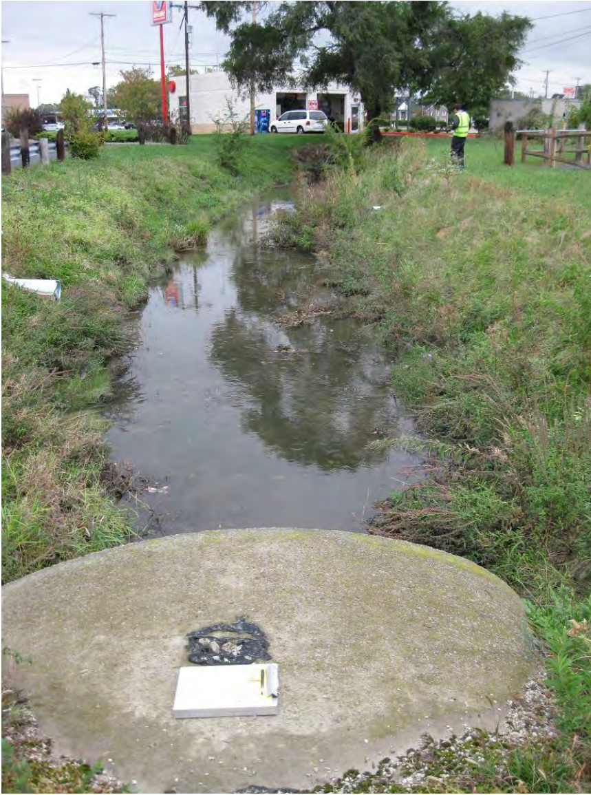
Amlosch Ditch Photo 6: Outfall pipes and culvert on Amlosch Ditch.
