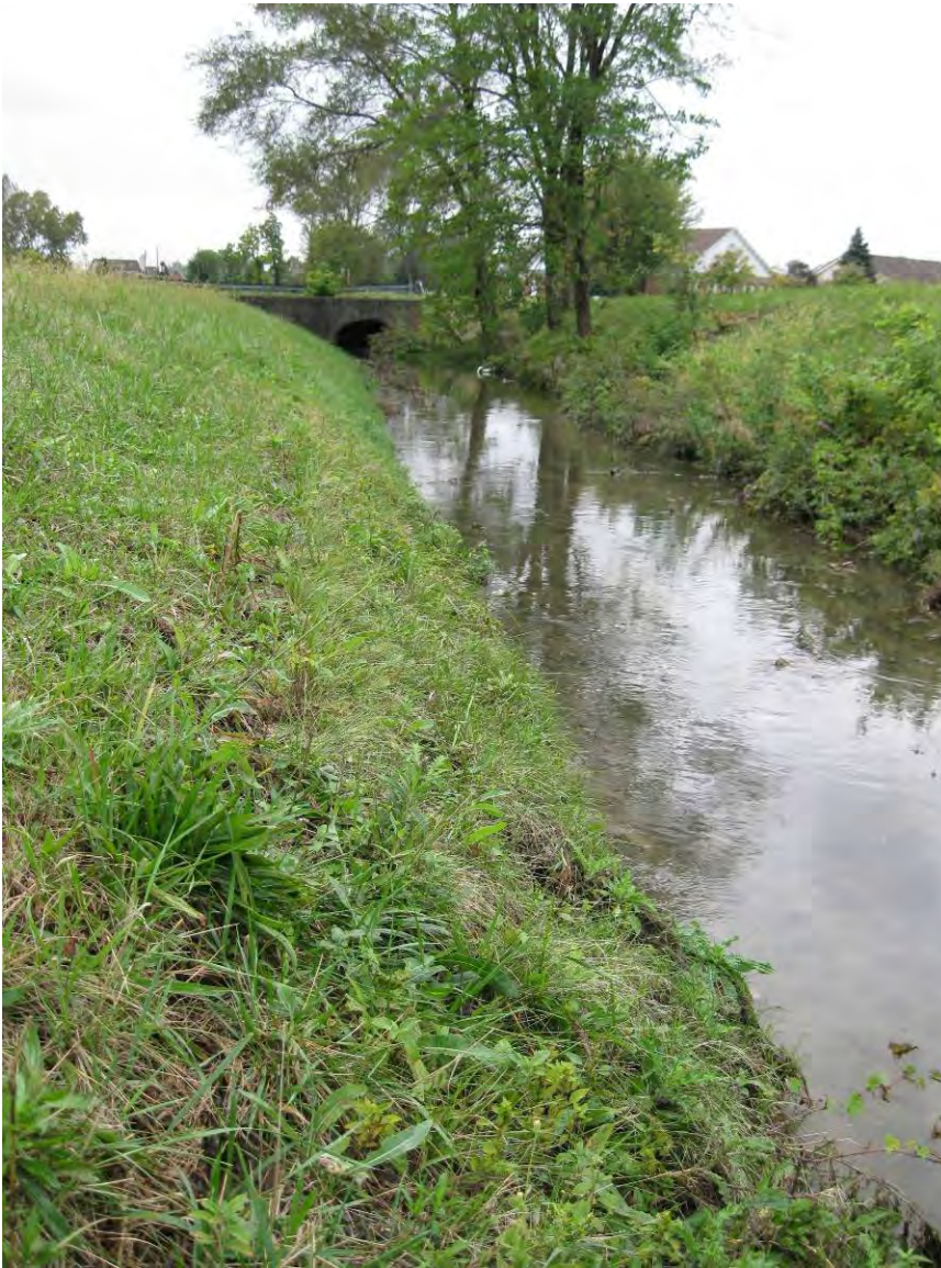
Amlosch Ditch Photo 3: Amlosch Ditch exhibiting lack of channel sinuosity.
