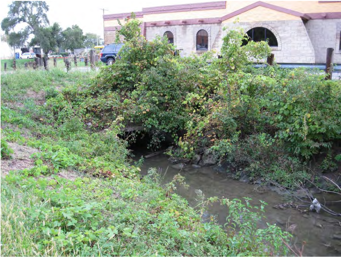
Amlosch Ditch Photo 1: Amlosch Ditch passing through culvert.
