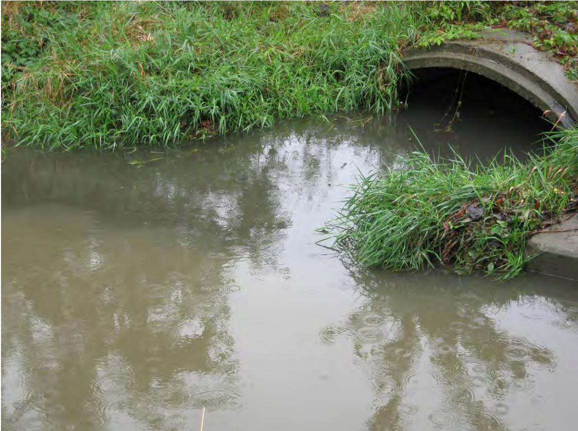
OC-22 Photo 3: Large outfall pipe along Otter Creek.
