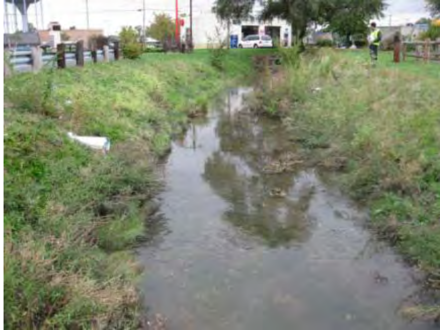
Figure 3-6 Sample station in Amlosch Ditch (AD-1), depicting little to no bank erosion, high channel stability and little to no instream cover.
