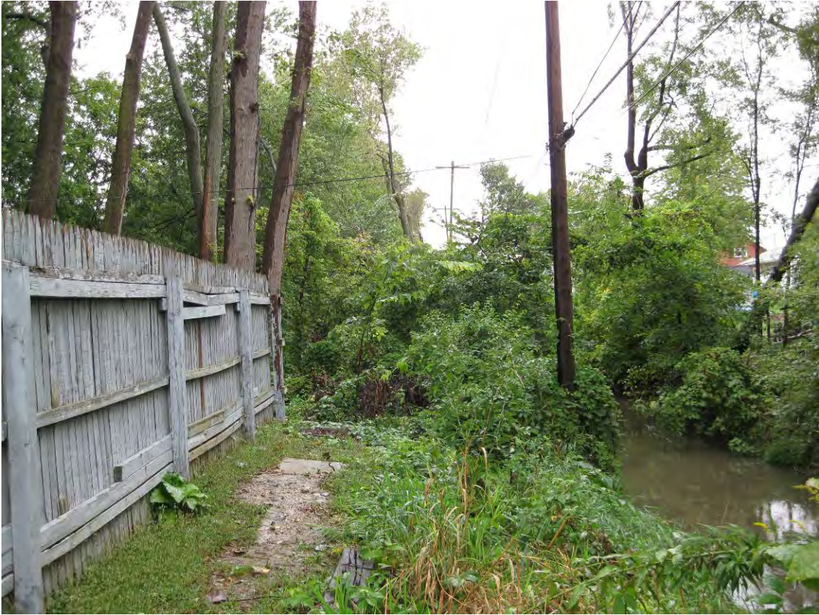
OC-22 Photo 10: Otter Creek segment with residential flood plain.
