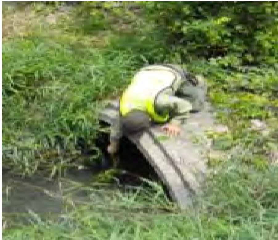
Figure 3-20 A large stormwater outfall enters Otter Creek from the east bank near OC-22 in Segment D.
