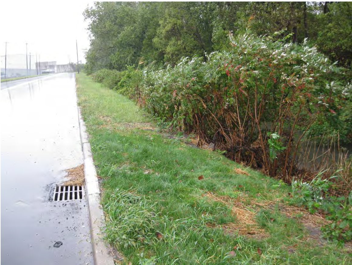
DC-3 Photo 3: Stormwater drain along Duck Creek.
