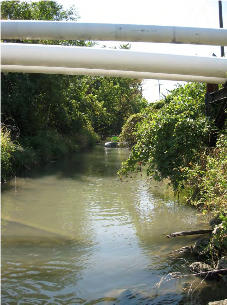
OC-6-7 Photo 4: Otter Creek segment exhibiting woody debris and boulders.
