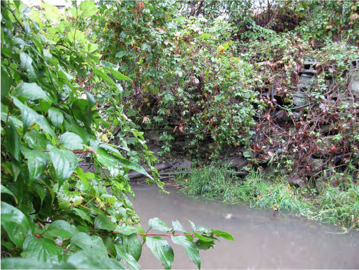
OC-22 Photo 7: Rock wall along Otter Creek.
