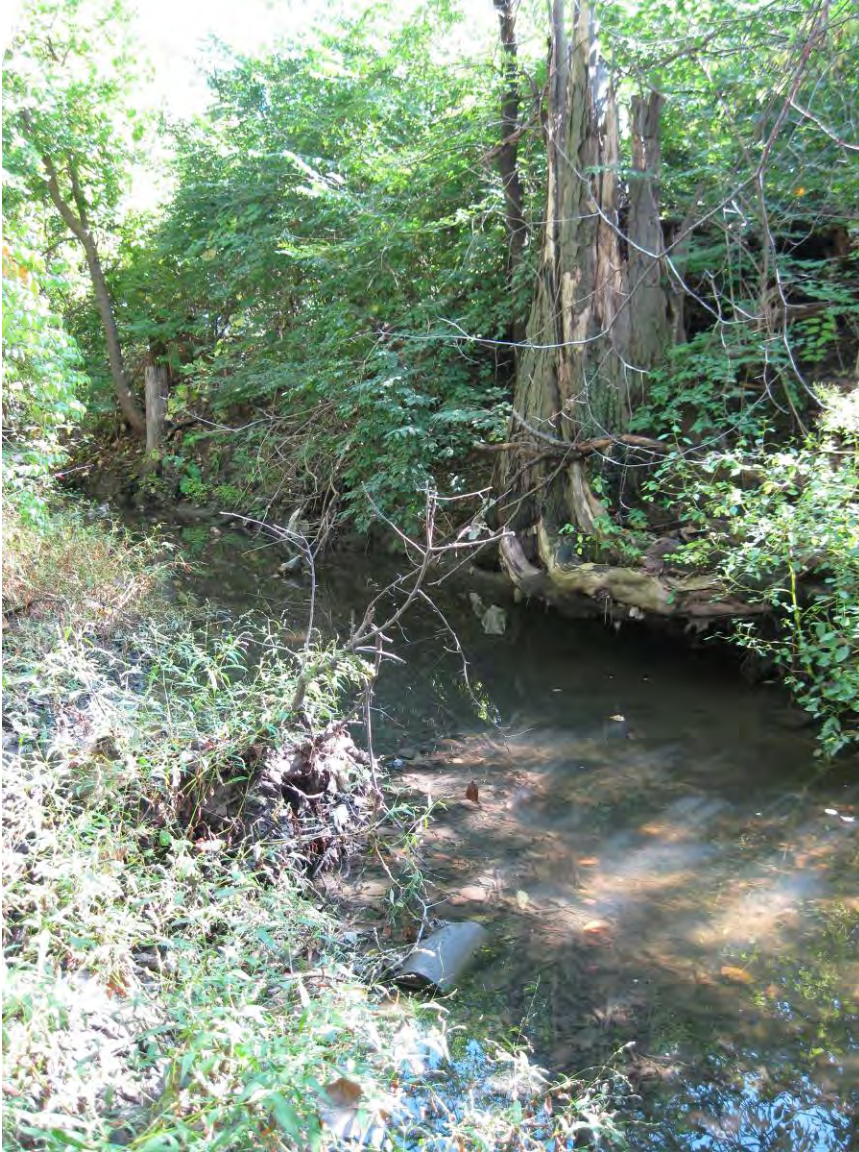
Grassy Creek Photo 9: Undercut bank along Grassy Creek.
