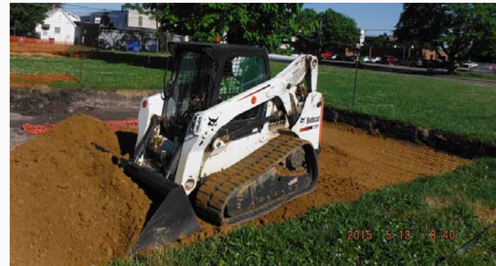
Skid-steer (Backfill placement)
