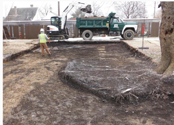
Surficial soil removed under tree canopy
