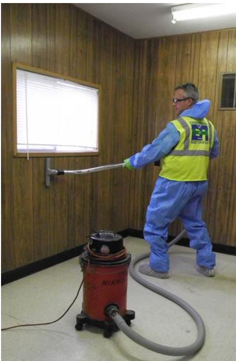
This photo shows what cleaning crews will wear inside your home and the vacuum they will use. These are EPA contractors from the company Environmental Restoration, managed by EPA.
