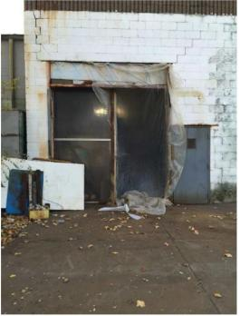
Photo 41: Missing bay door on north side of building
