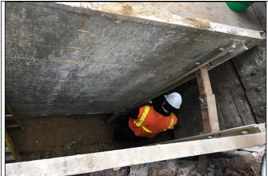
Photo 3: View of screening excavation sidewalls and floor
