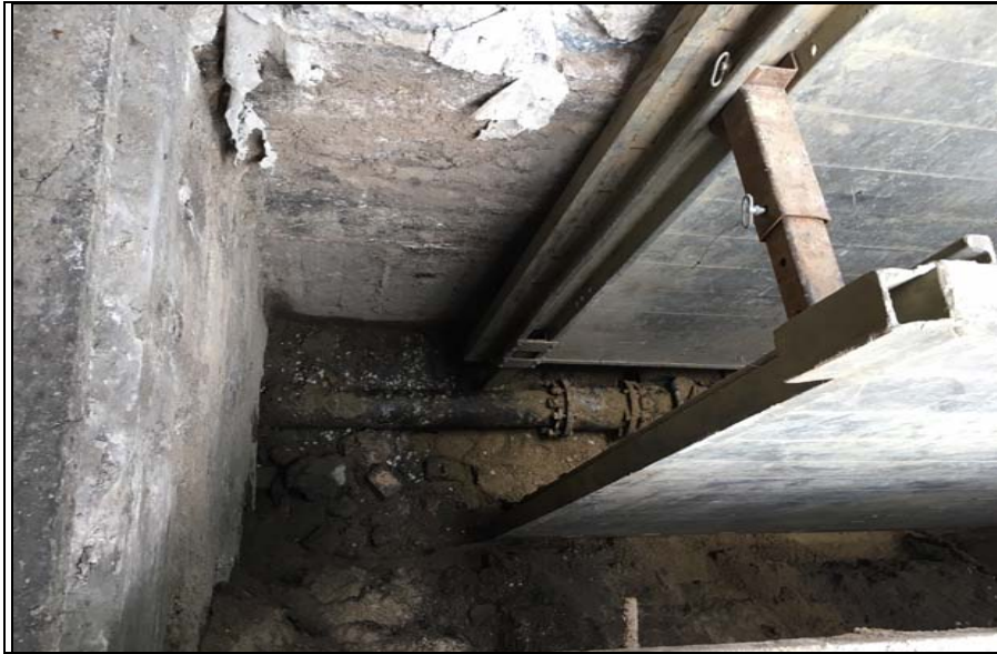
Photo 1: View of water main replacement
