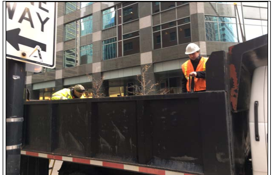
Photo 4: View of screening excavation soil spread out on floor of dumptruck
