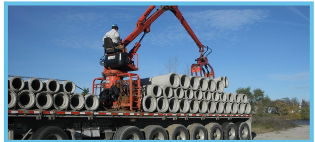
Concrete pipes for drainage culverts under new gravel road
