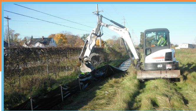
EPA begins site preparation work at the Velsicol site. See page 1 for details.
