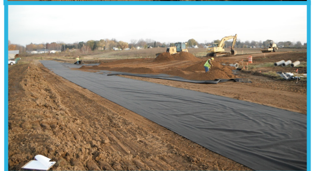
Workers construct new haul road to support cleanup of Main Plant site
