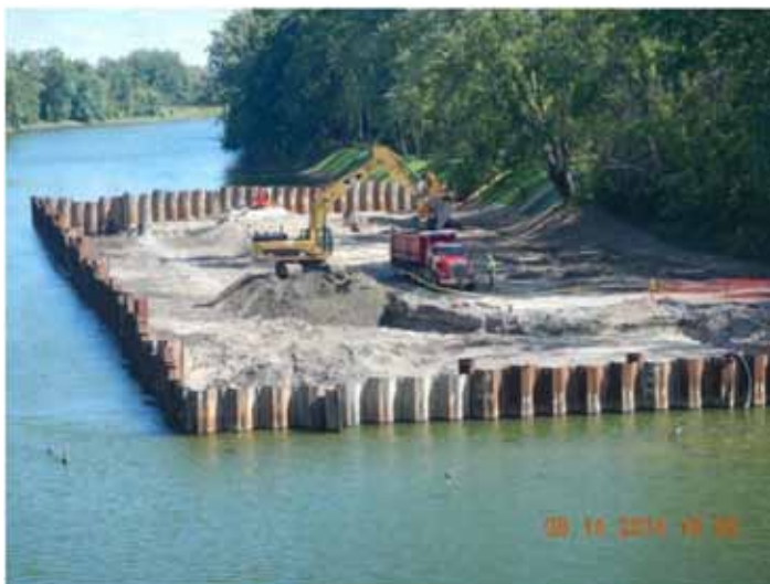
Removing sediment in dry conditions.
