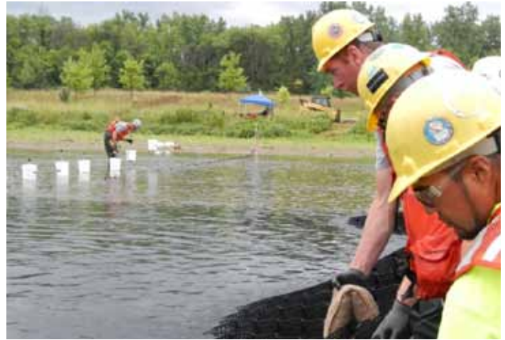
Workers install a CCS cap.
