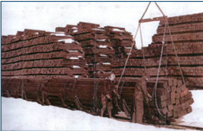
Workers unloading railroad ties.
