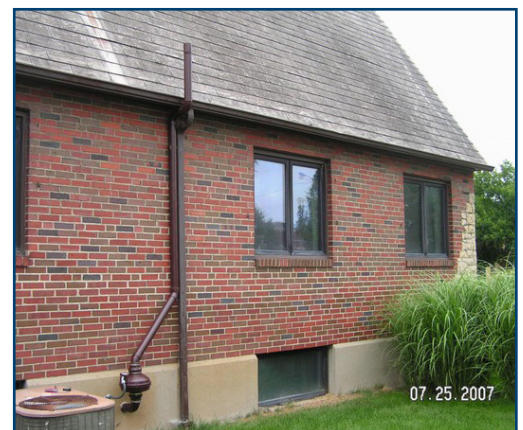
A vapor removal system on a home.
