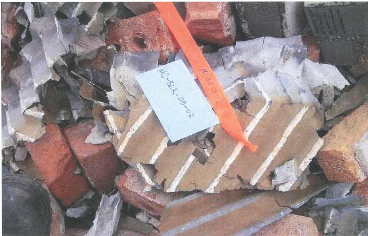
Corrugated paper tested positive for asbestos
