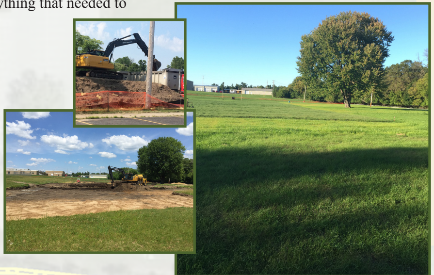
Work to remove DDT-contaminated soil in areas of St. Louis Public Schools' Athletic fields.
