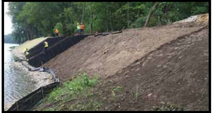
Workers stabilizing a bank in Segment 2.
