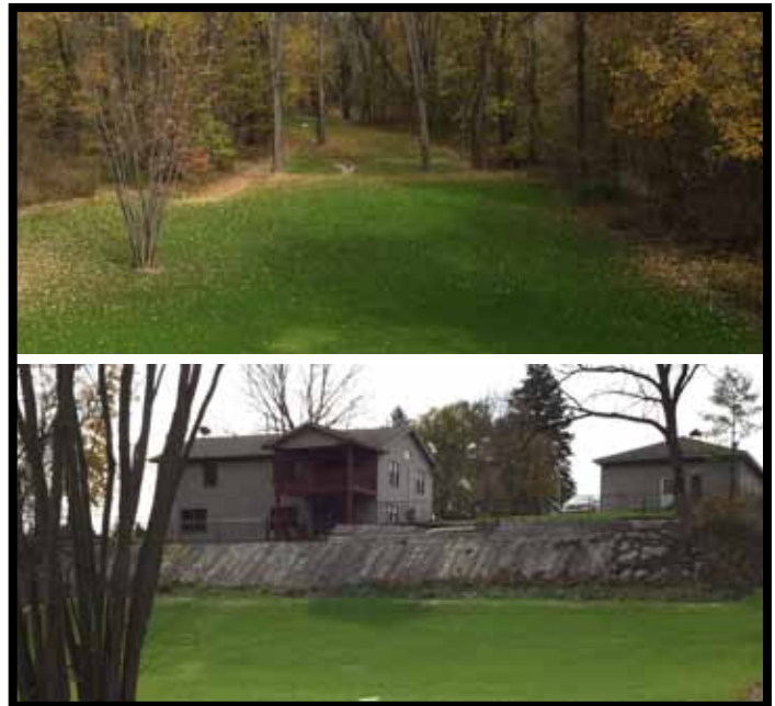
Work completed and grass reestablished in yard.
