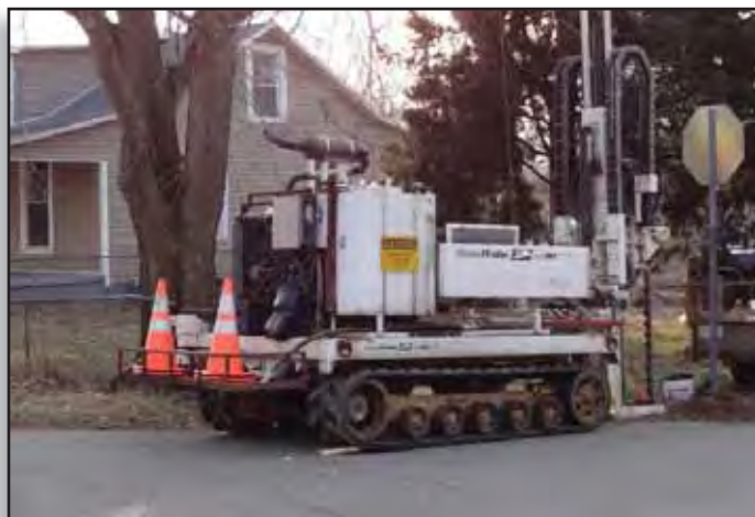
U.S. EPA installed and sampled 13 temporary groundwater wells in the Riverside neighborhood.
