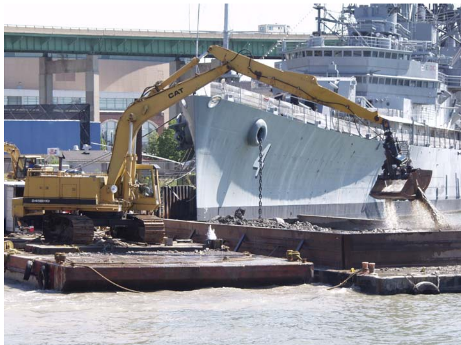
BIDCO removing “shot-rock” it blasted to make way for USS Littlerock
