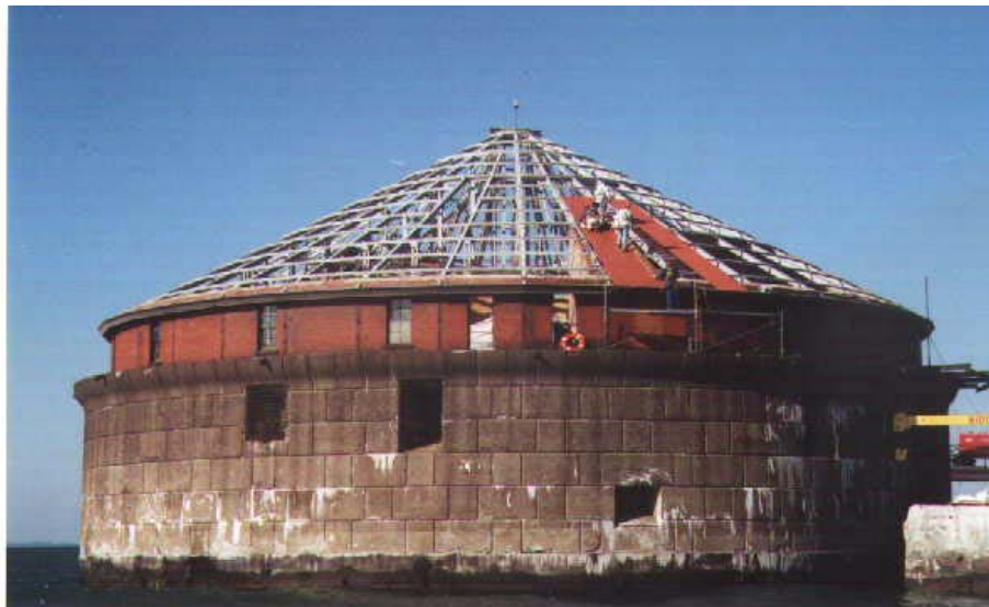
BIDCO Crew installing roof panels at "Round-House"
