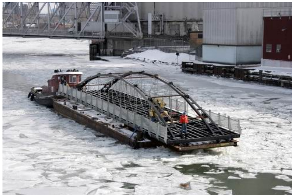
BIDCO vessels delivering completed "Whipple Truss Bridge" to Erie Canal
