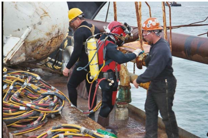
BIDCO Diver & Tenders working on Northeast Gateway Pipeline/Offshore LNG Terminal
