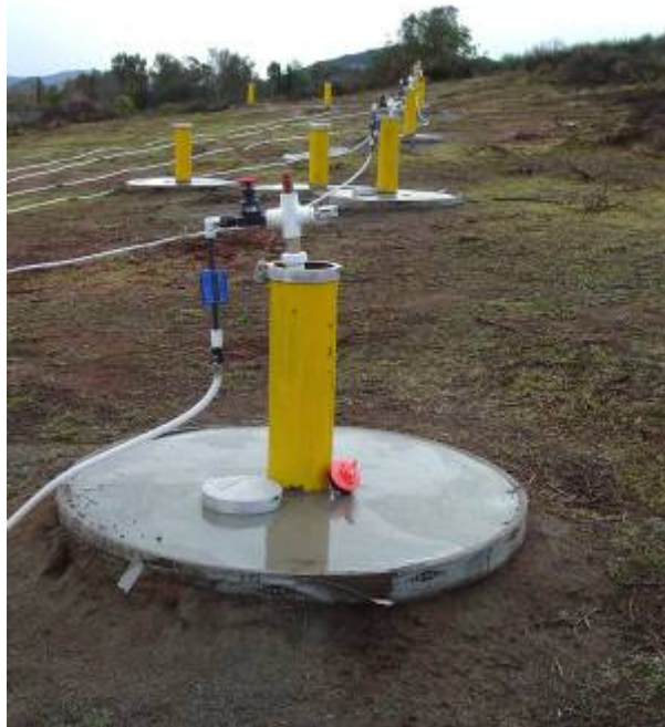
Figure 5.9 Typical Well Head Configuration (Photo courtesy of Remediation and Natural Attenuation Services, Inc.)
