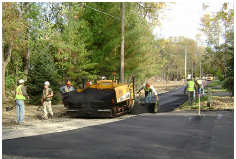
Covering road with new asphalt.
