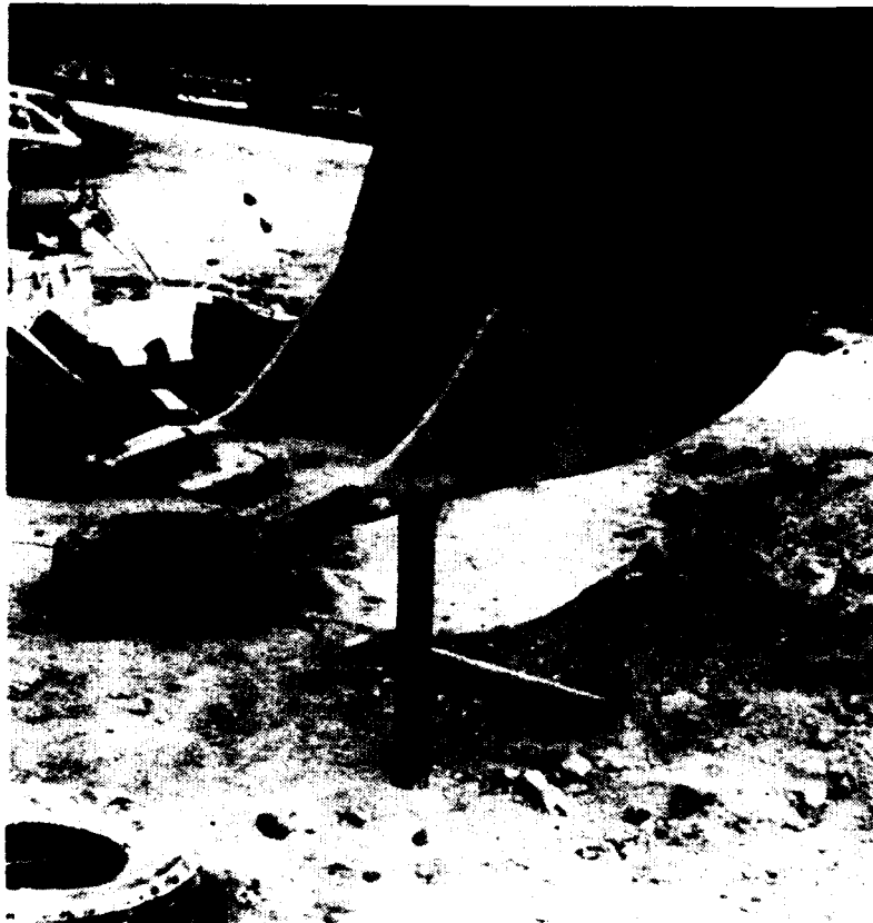
Figure 6-11. Pushing of thin-walled sampling tube with a backhoe.
