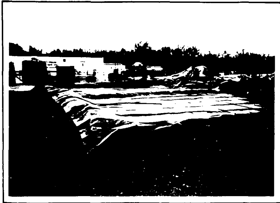
① PVC LINER FOR BERMED STAGING PADS. POTABLE AND WASHWATER STORAGE TANKS IN BACKGROUND - DECEMBER 5, 1989
