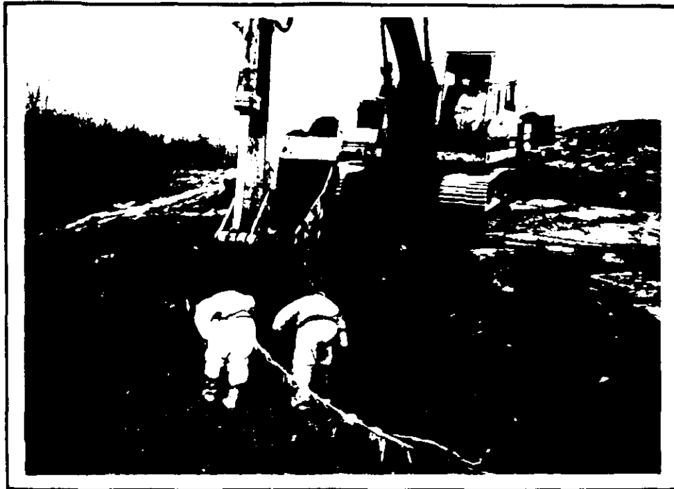
30 DRUM REMOVAL AT SUPPLEMENTAL NEBD AREA - JANUARY 29, 1990
