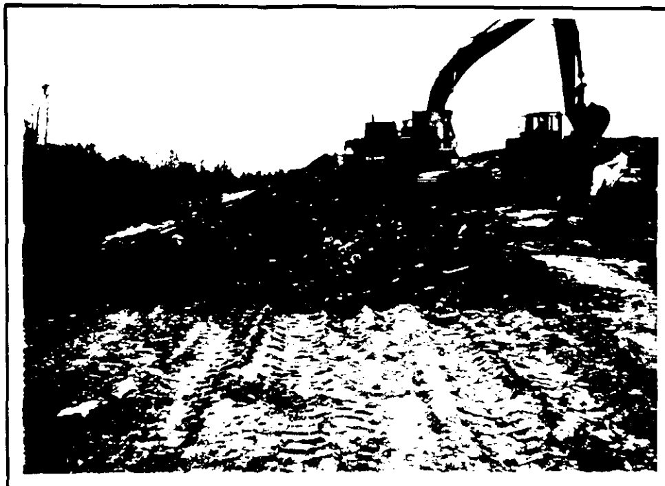
32 COMPLETED EXCAVATION AT NEBD AREA (LOOKING SOUTH) - JANUARY 29, 1990
