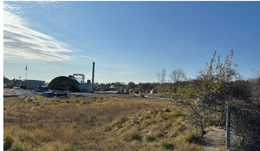
In situ soil treatment operations.
