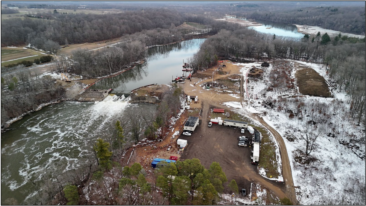
Trowbridge Staging Area with the dam in view, where crews stage equipment and materials for ongoing river cleanup.
