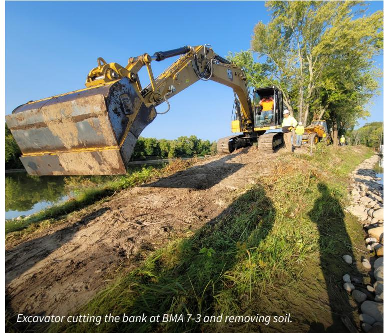
*Excavator cutting the bank at BMA 7-3 and removing soil.*
