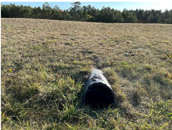
Photograph 5: OU2 Surface water runoff conveyance pipe
