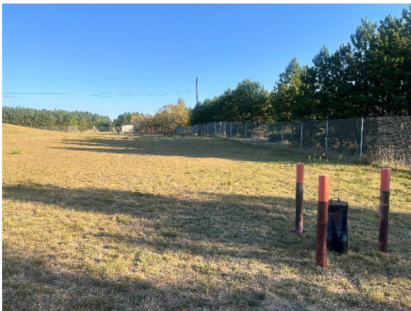
Photograph 23: OU2 east side looking north toward force main shed
