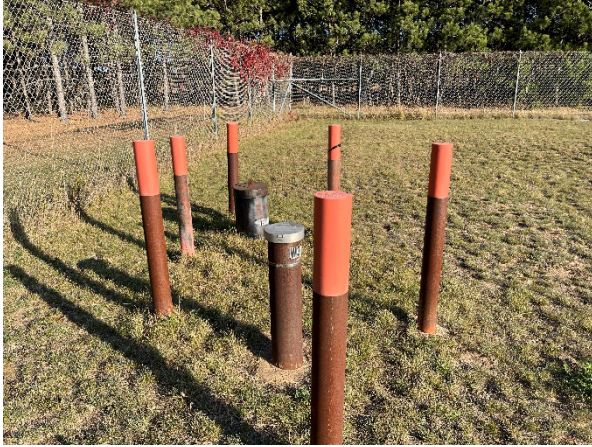
Photograph 21: OU2 monitoring well W324 (looking north)
