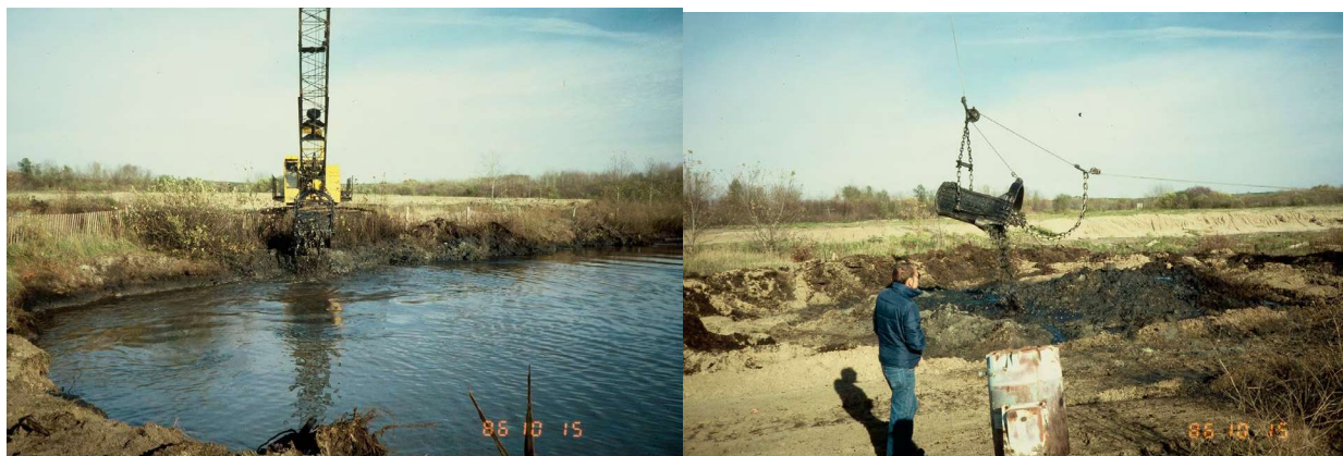
Photos show a bucket dredge removing sludge from an OUI waste pond in 1986. The ponds were not drained and were backfilled with contaminated soil from OU2.
