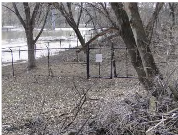
The MAC traverses the SARL site to access the northern end of the stormwater detention pond
