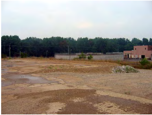
View southwest towards the city's wastewater treatment plant and concrete slabs that cover a majority of the southern portion of the site.
