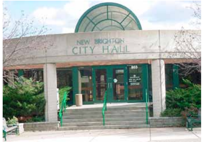
The City of New Brighton's acquisition of the MacGillis & Gibbs property in 1997 enabled cleanup and redevelopment to move forward.
