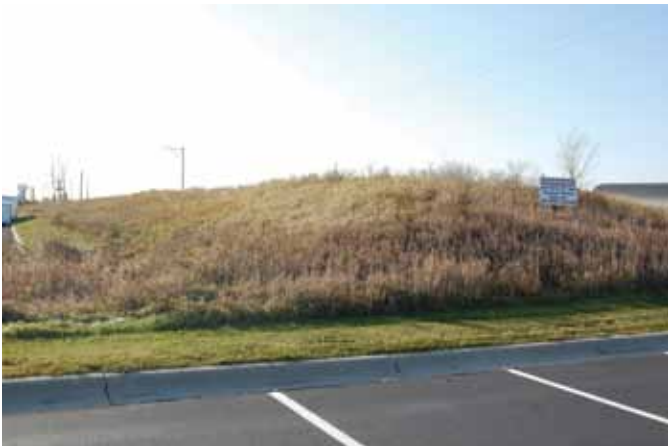
Capped and vegetated soil containment area on the site.
