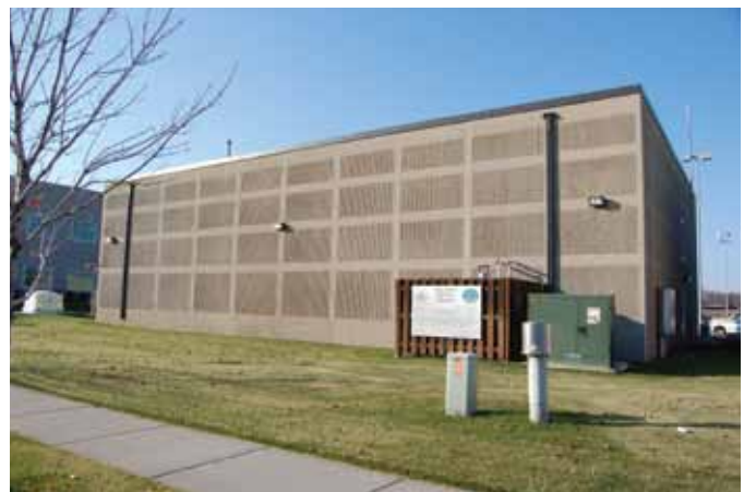
Ground water treatment facilities on the site property.
