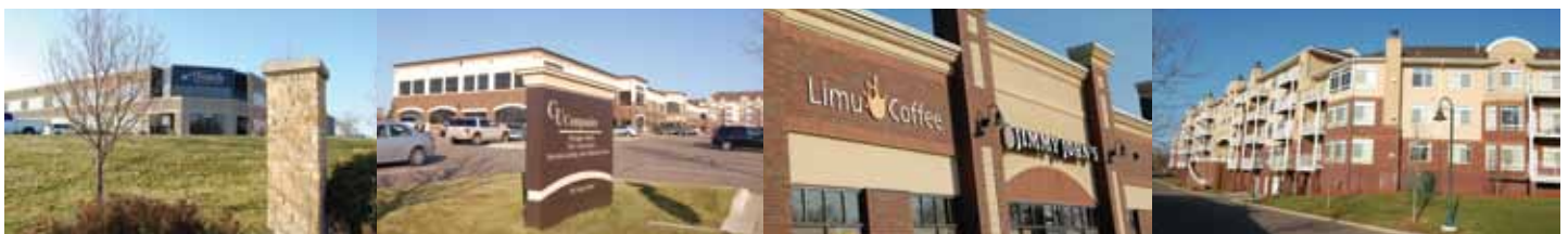
Manufacturing, commercial office, commercial retail and residential land uses at New Brighton Corporate Park III, 2010.
