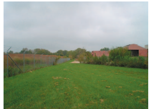
View of the consolidation area and warehouse buildings
