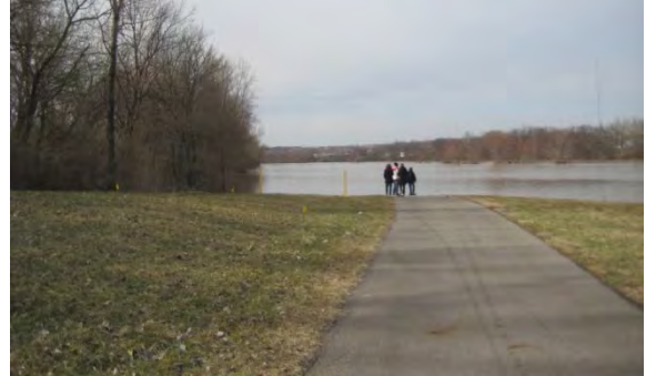
The Great Miami River and Great Miami River Recreation Trail are adjacent to the Site. At the time of the site visit, recent rains had caused the river to cover parts of the trail.
