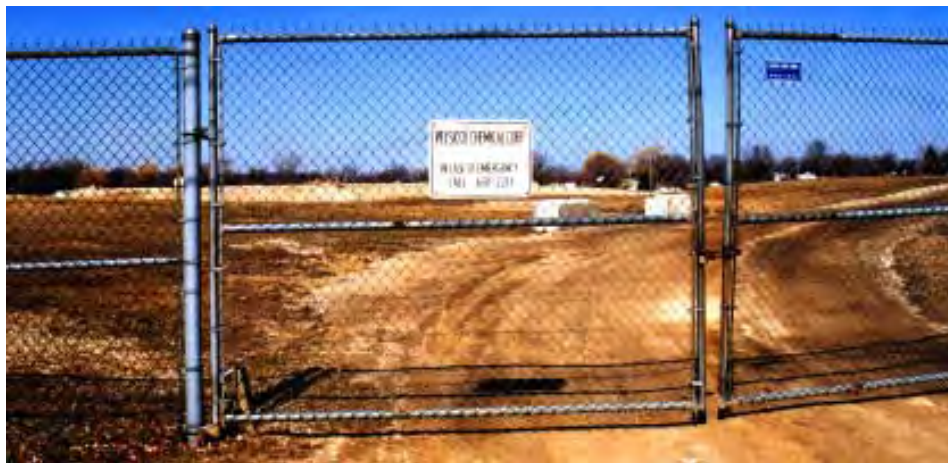
Existing Entry Gate to the Velsicol Chemical Corp. Superfund Site
