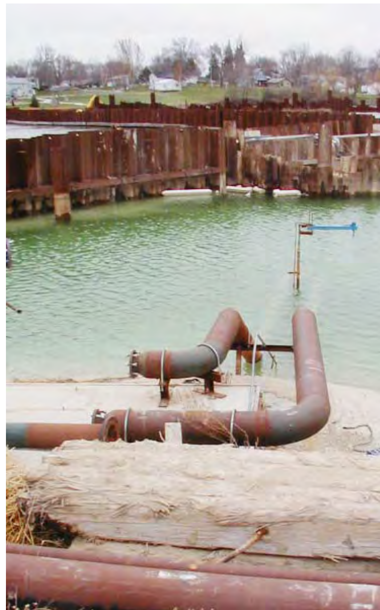
Dewatering Cells in the Pine River (2003)
