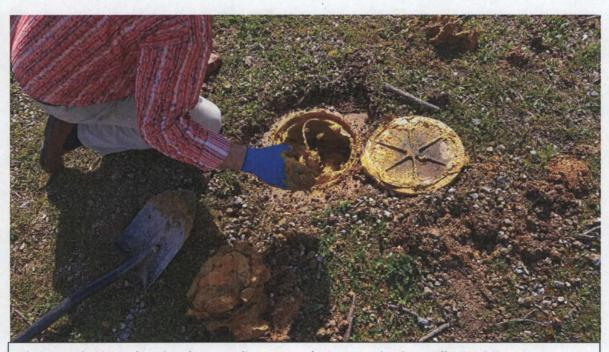
Photograph 13: Unburying downgradient groundwater monitoring well MW-24i.
