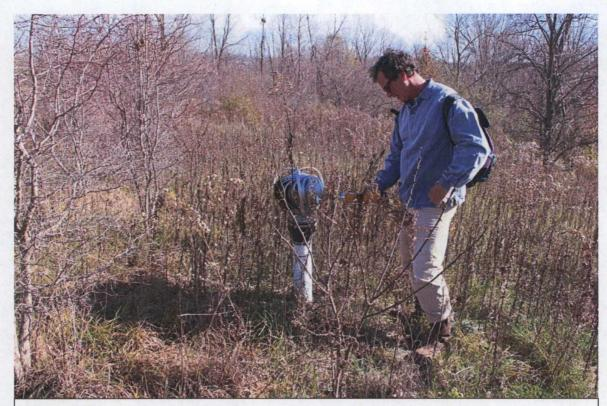
Photograph 6: Unlabeled passive gas vent venting about three (3) feet off the ground.
