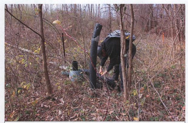
Photograph 8: Unlabeled pipes of unknown construction venting gas in northeast area of Site near EW-12.
