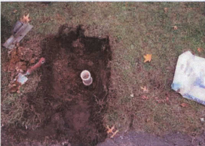
Concrete pad replacement for MW-34
