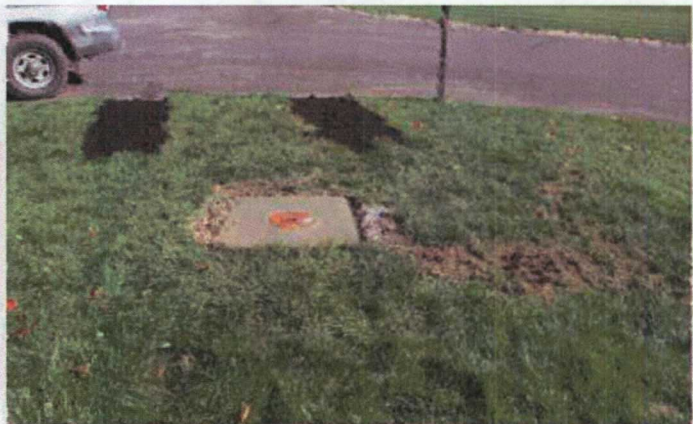
Flush mount concrete pad for MW-45 (view east)
