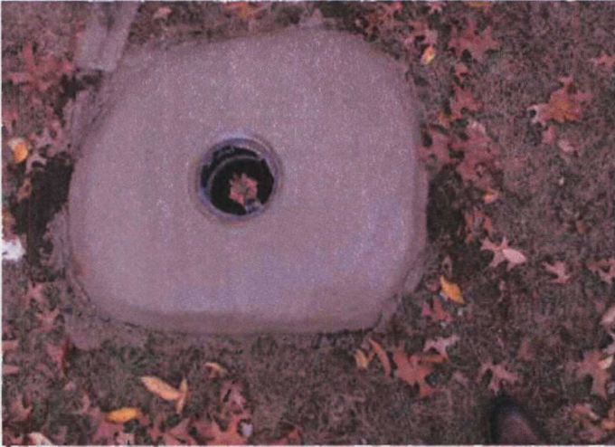
11/07/2013: Maintenance to flush mount pad for MW-16.
