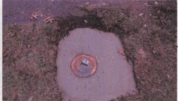
11/07/2013 Maintenance to flush mount pad for MW-27 and MW-28
