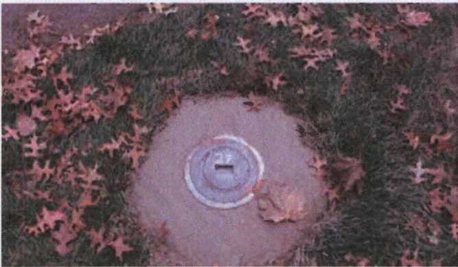
11/07/2013 Maintenance to flush mount pad for MW-27 and MW-28
