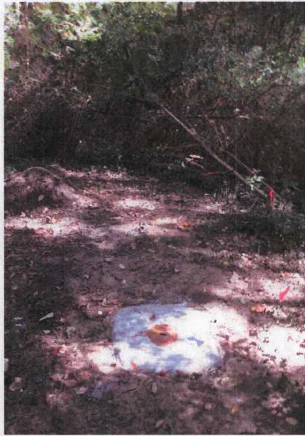
Flush mount concrete pad for MW-18R (view east)
