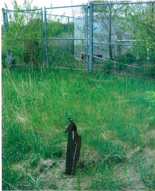
Picture 4 – Damaged Monitoring Well G120
