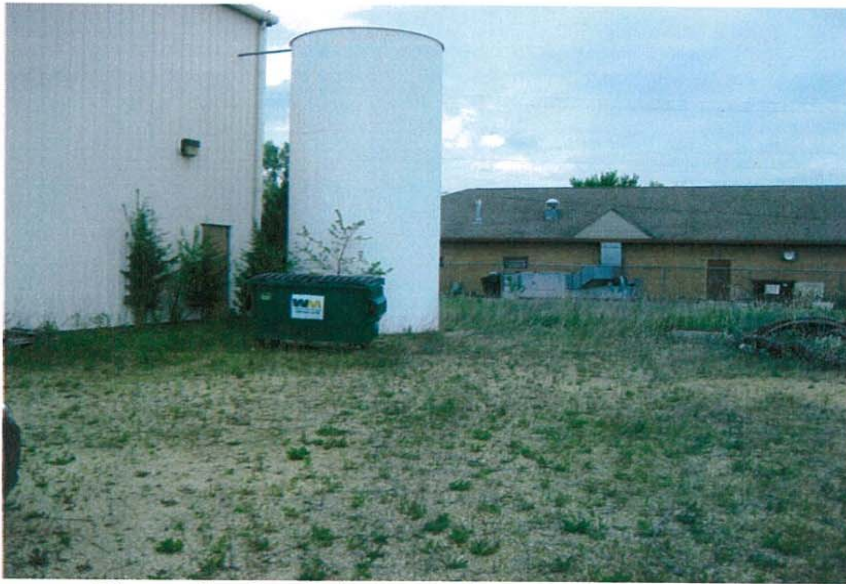
Picture 6 – General Site conditions within the fence
