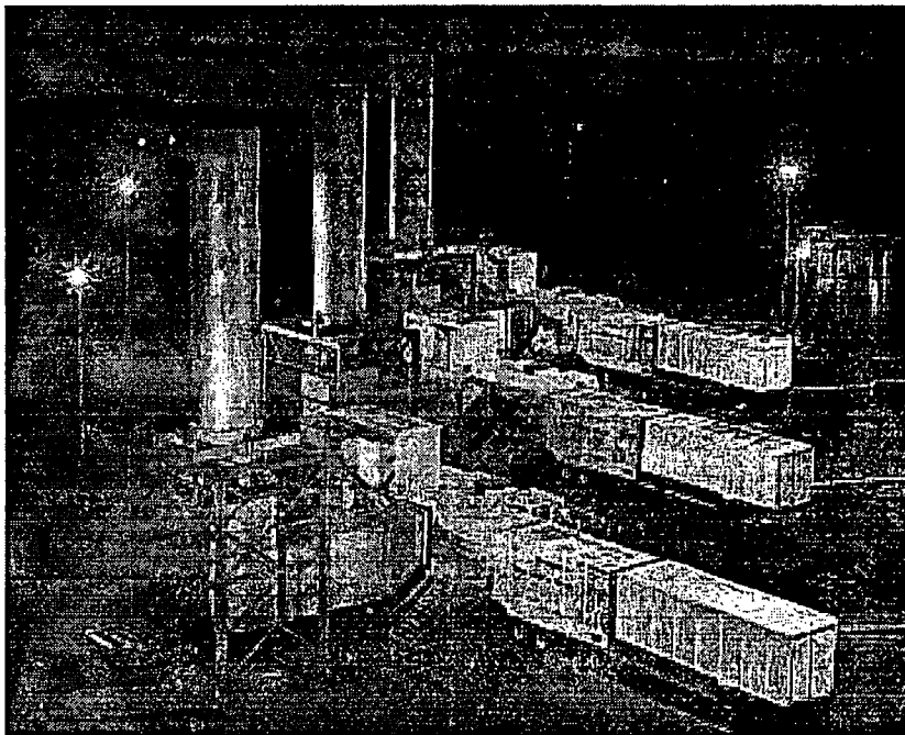
This trailer-mounted Power Plant on Wheels is located in Cork, Ireland. These 22.8 megawatt units are more fuel-efficient and more environmentally friendly and occupy less space than other temporary power solutions.
