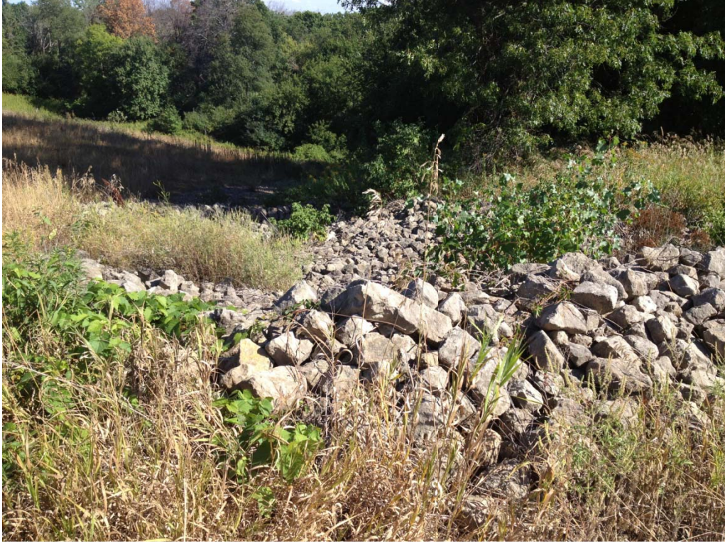
Site 129-15, Rip rap for mitigation of run-off from upper road
