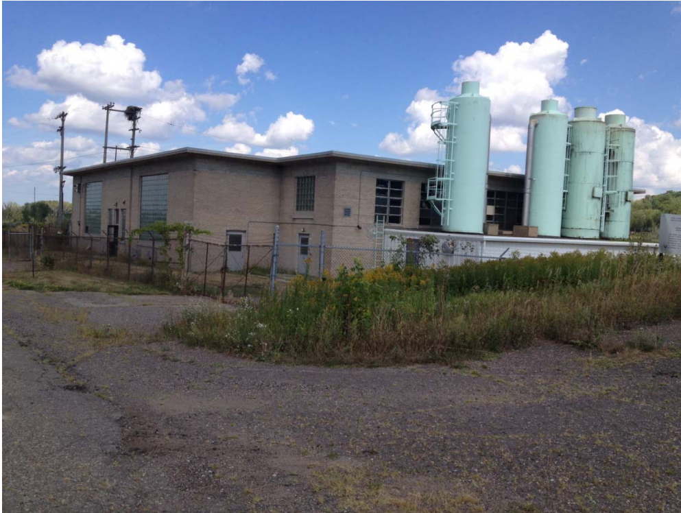
TCAAP Groundwater Recovery System
