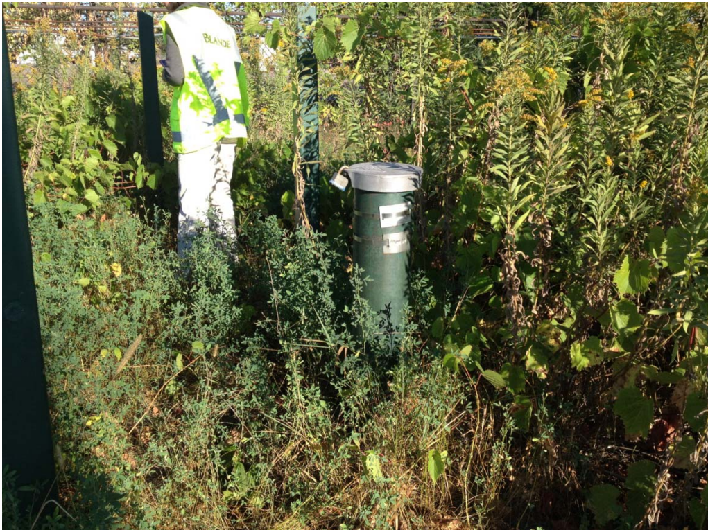
Site K, Monitoring Well 03U621. Good condition and well marked.
