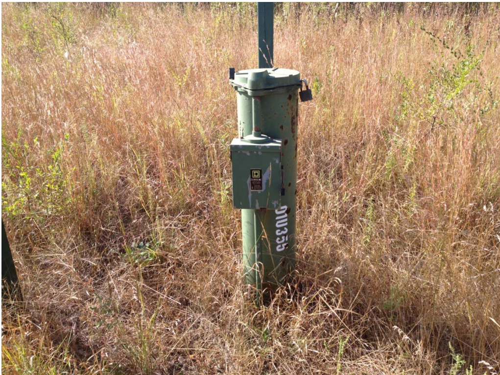
Site A, Monitoring Well 01U355. Good condition and well marked.
