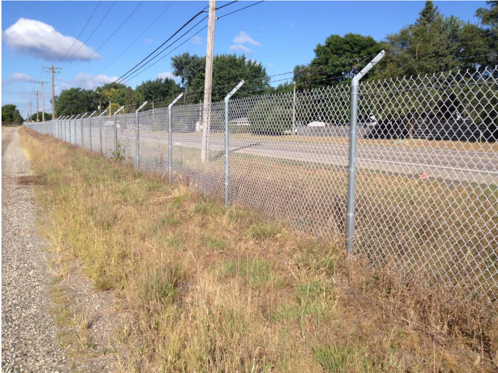
Site A, Example of Perimeter Fence
