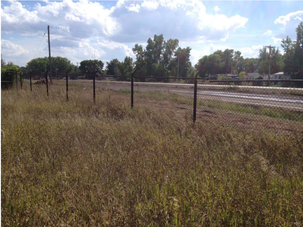
TCAAP Perimeter Fence, adjacent to Relief Well B-6 Pump House
