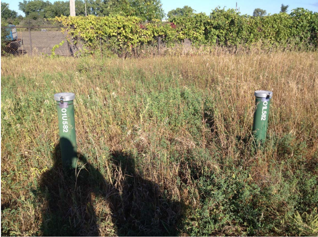
Site 102, Monitoring Well 01U582 and 01L582. Good condition and well marked.
