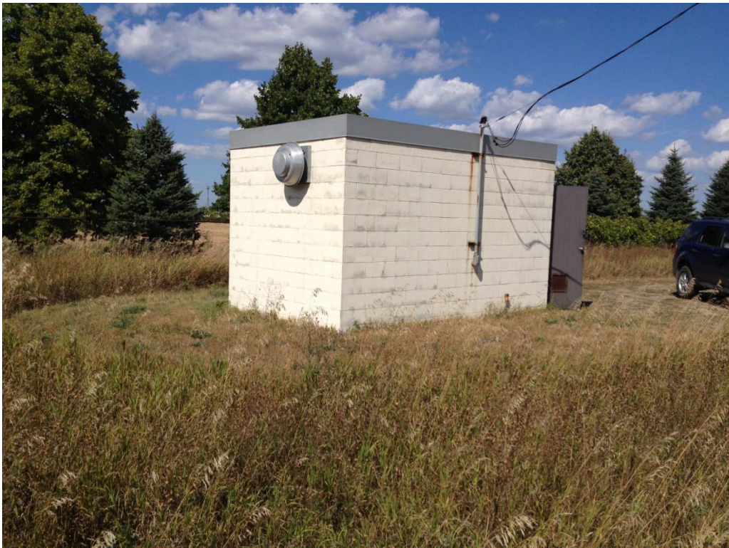
Relief Well B-6, Pump House
