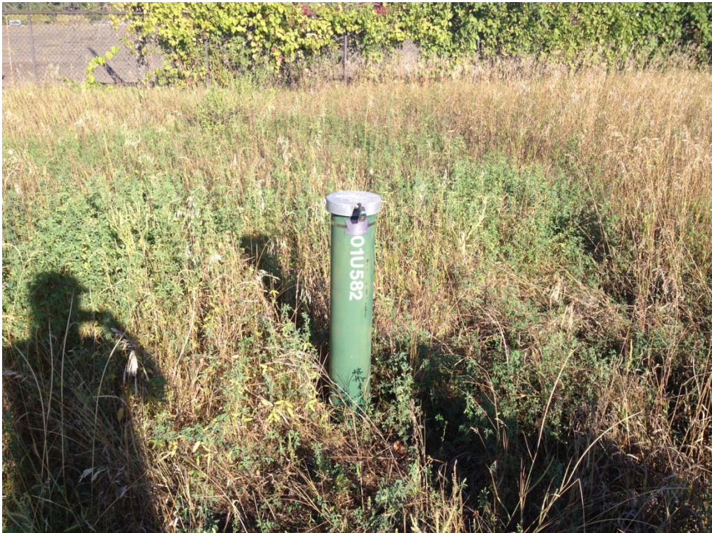
Site 102, Monitoring Well 01U582. Good condition and well marked.
