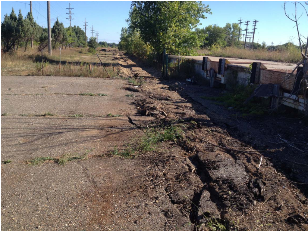
Site 102, Collection Trench
