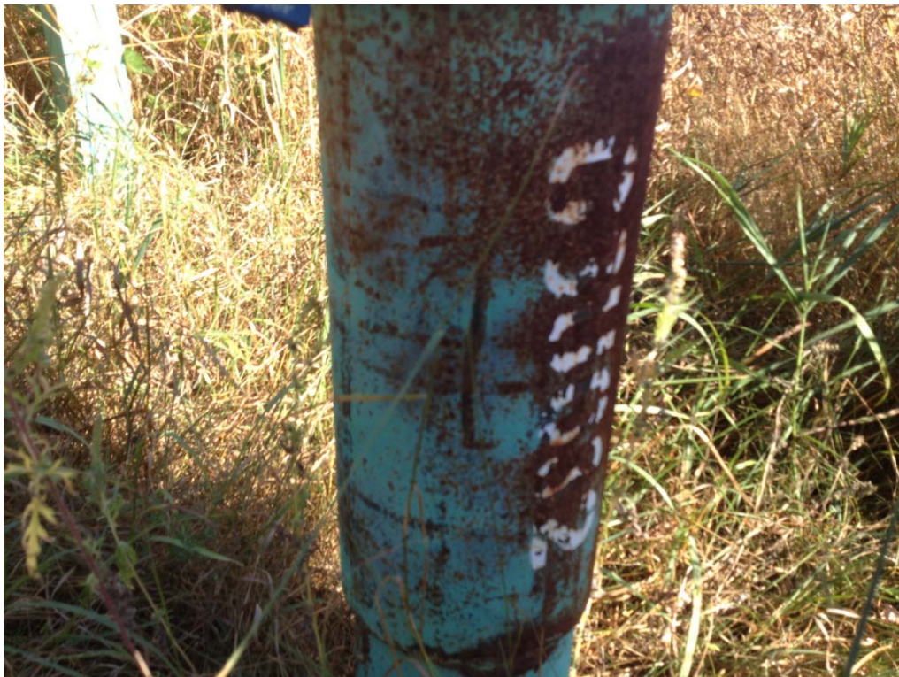
Site 129-15, Monitoring Well. Uncertain of well ID. Well may need to be abandoned.
