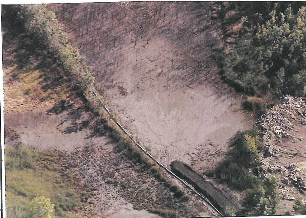
Discharge of zinc oxide to wetlands and Long Lake, 1996.
