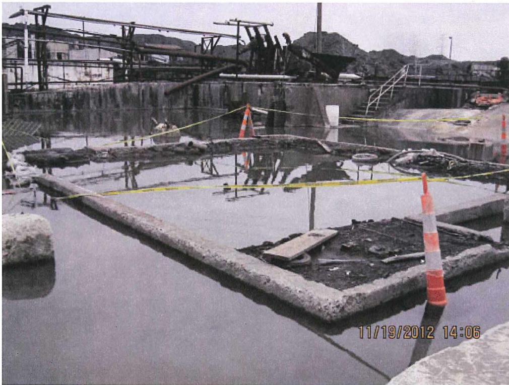
Flooding at Chemetco site, 2012.
