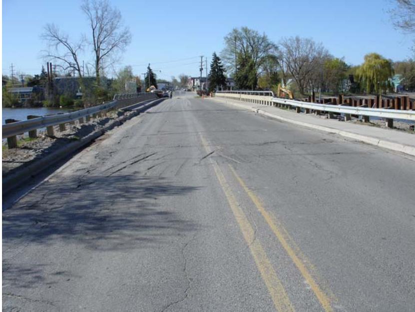
Photograph 1 - Looking South along structure
