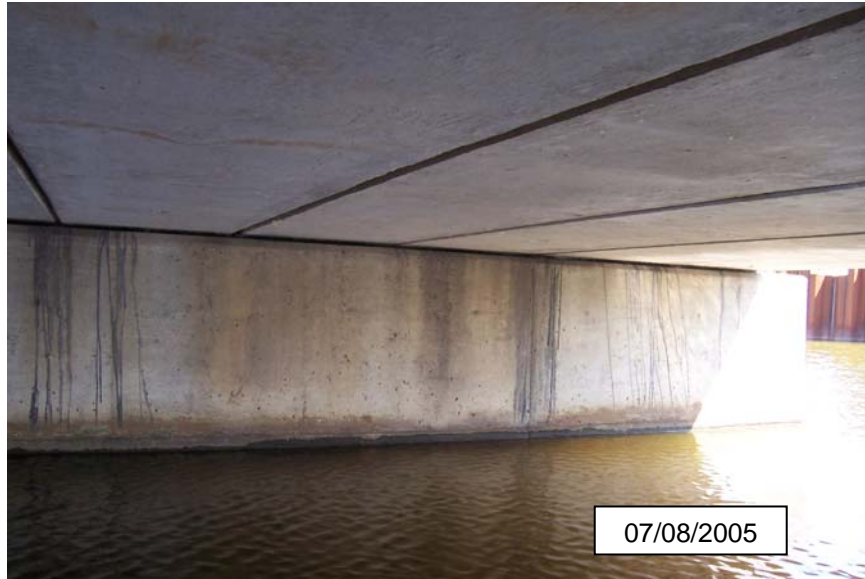
Photograph 17 - Beams at Span 1
