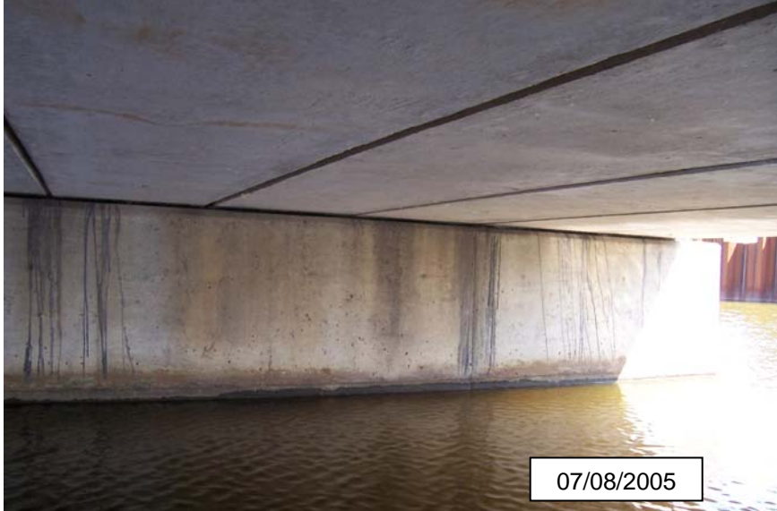
Photograph 16 - South face of Pier 1
