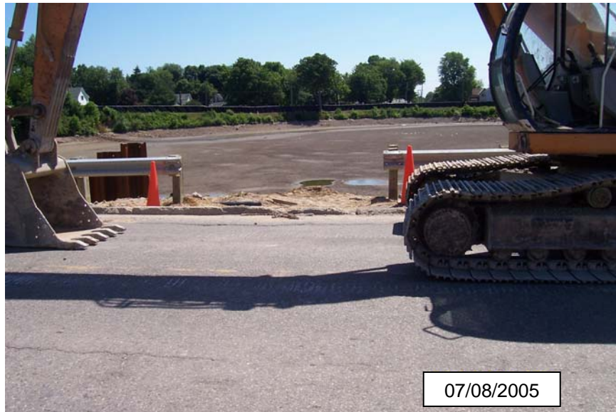
Photograph 20 - Northeast curb and guardrail removed
