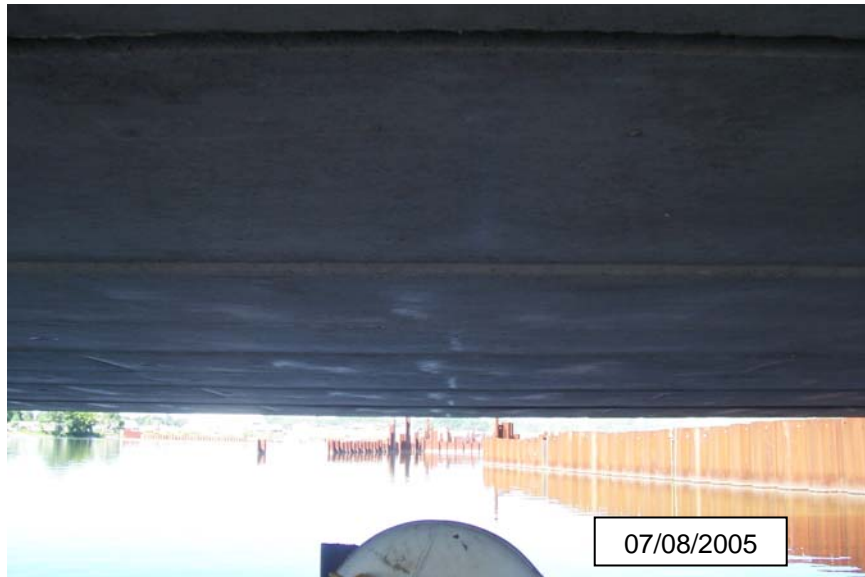
Photograph 14 - Beams at Span 2
