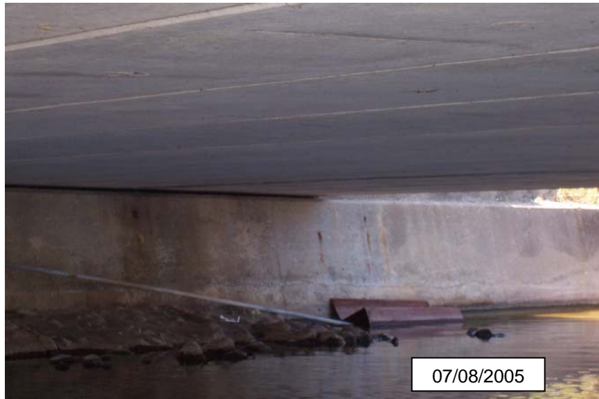
Photograph 18 - Face of South Abutment (west side)
