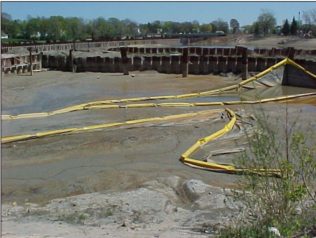
PHOTO 2—The equalization basin in April 2006 prior to its removal.
