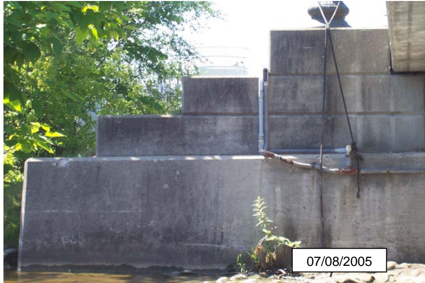
Photograph 19 - Face of South Abutment (east side)
