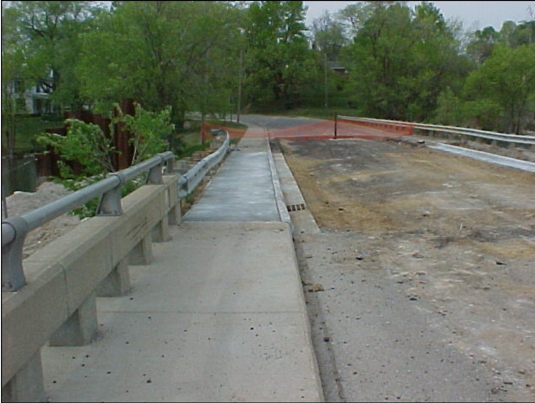
PHOTO 7—Previously damaged sidewalk after replacement in May 2006.
