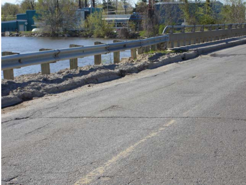
Photograph 5 - Northeast curb and guardrail removed
