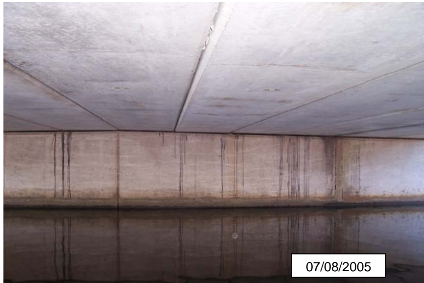
Photograph 12 - North Face of Pier 2
