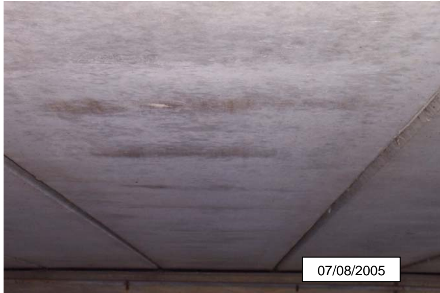
Photograph 11 - Interior beam at Span 3
