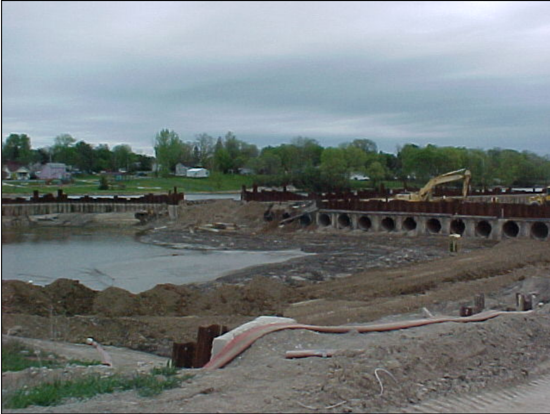
PHOTO 5—Removal of the north/south haul road underway in May 2006.
