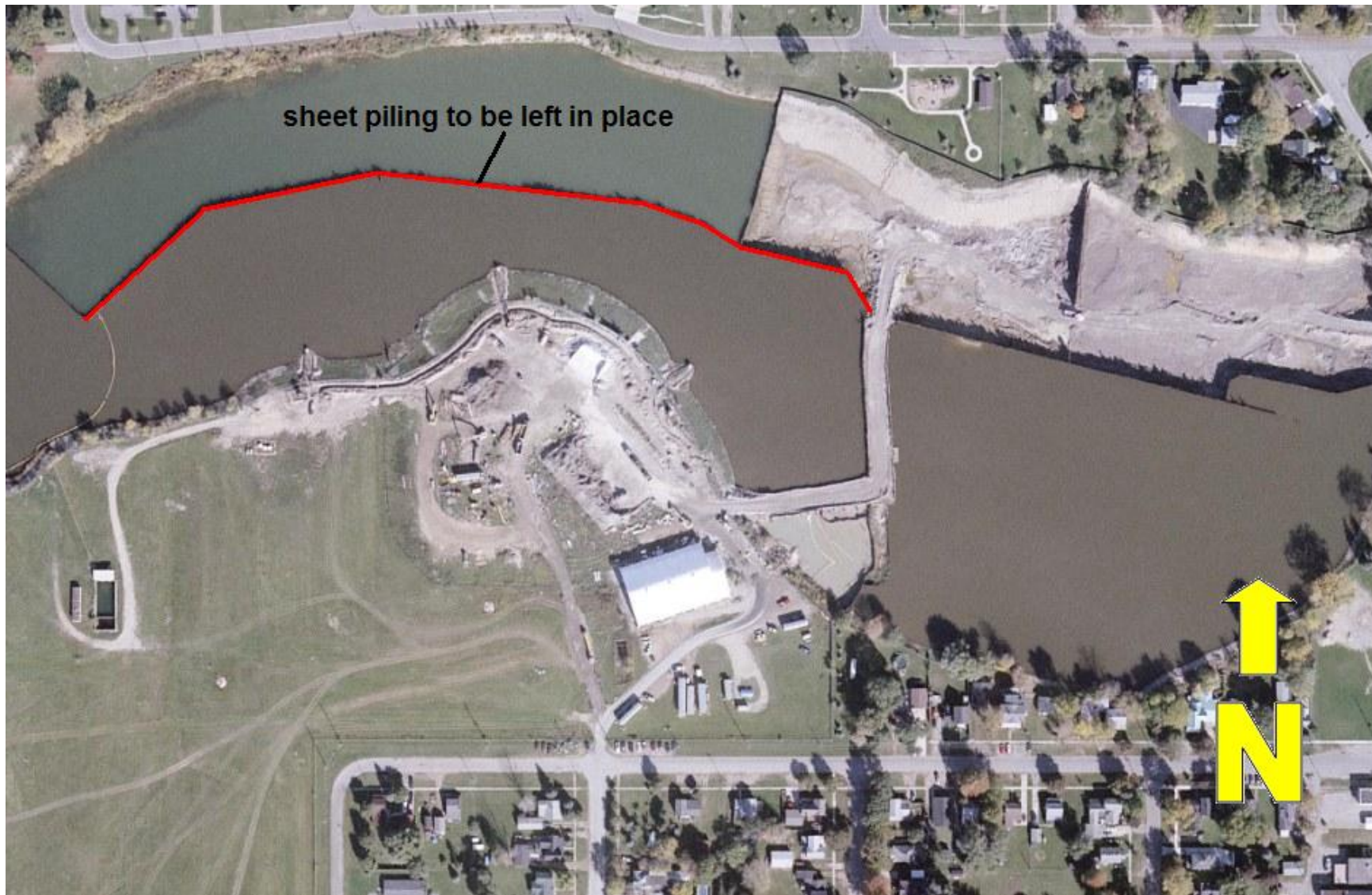
Figure 1. Sheet Piling Proposed to Be Left in Place Velsicol Chemical/Pine River Site in St. Louis, Michigan Proposal to leave 1480 LF of Sheet Piling in Place Memorandum
