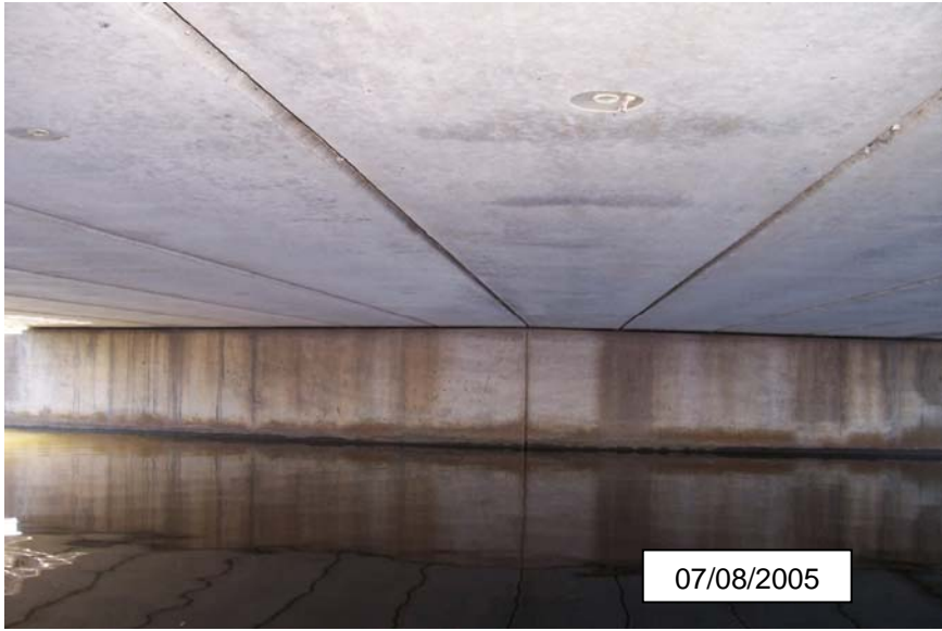
Photograph 15 - North face of Pier 1
