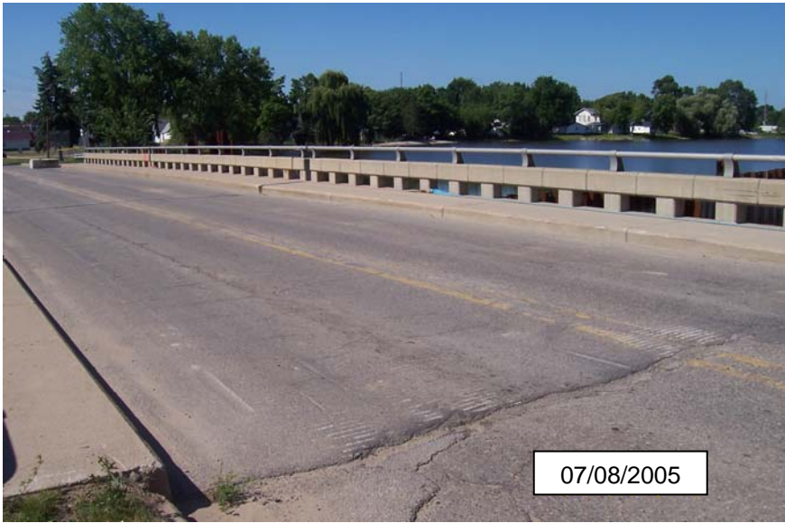
Photograph 1 - Looking South along structure
