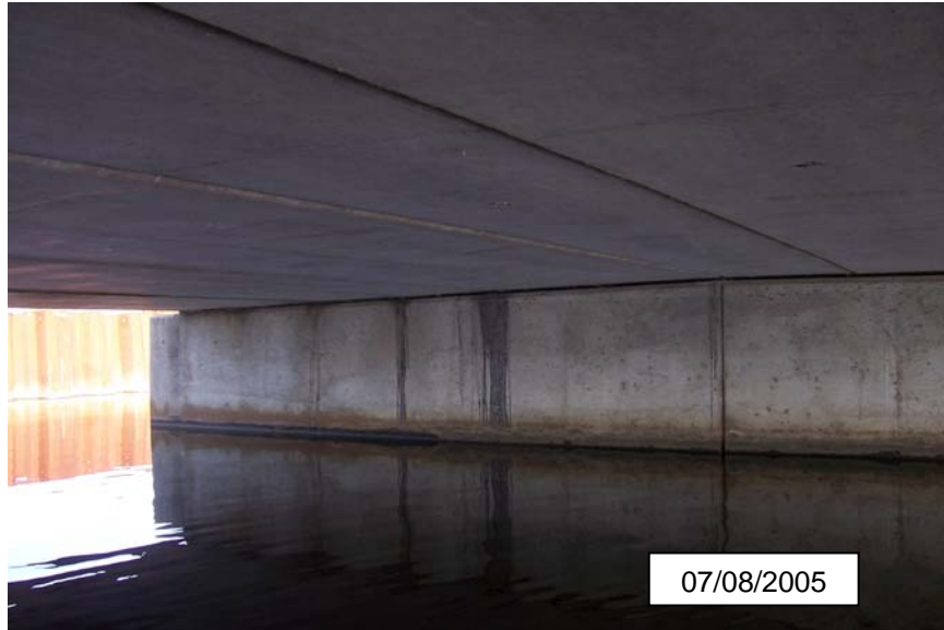
Photograph 13 - South face of Pier 2
