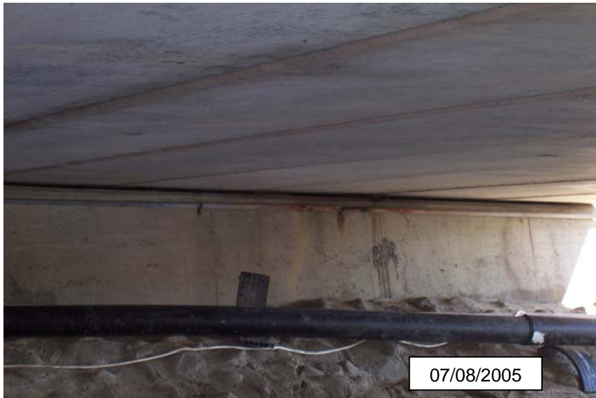
Photograph 10 - Face of North Abutment
